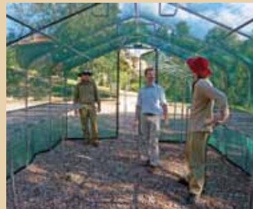
Coal Loader and Centre for Sustainability nursery shade house construction April 2011
