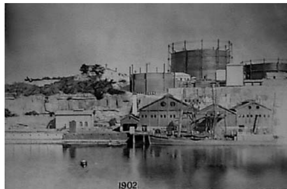
(North Shore Gas Company works, 1902. (Courtesy AGL)
