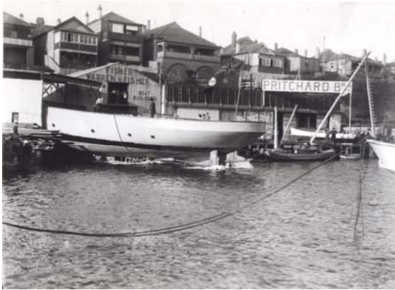
Boatsheds at Careening Cove, c. 1920s. (North Sydney Heritage Centre, PF 776)
