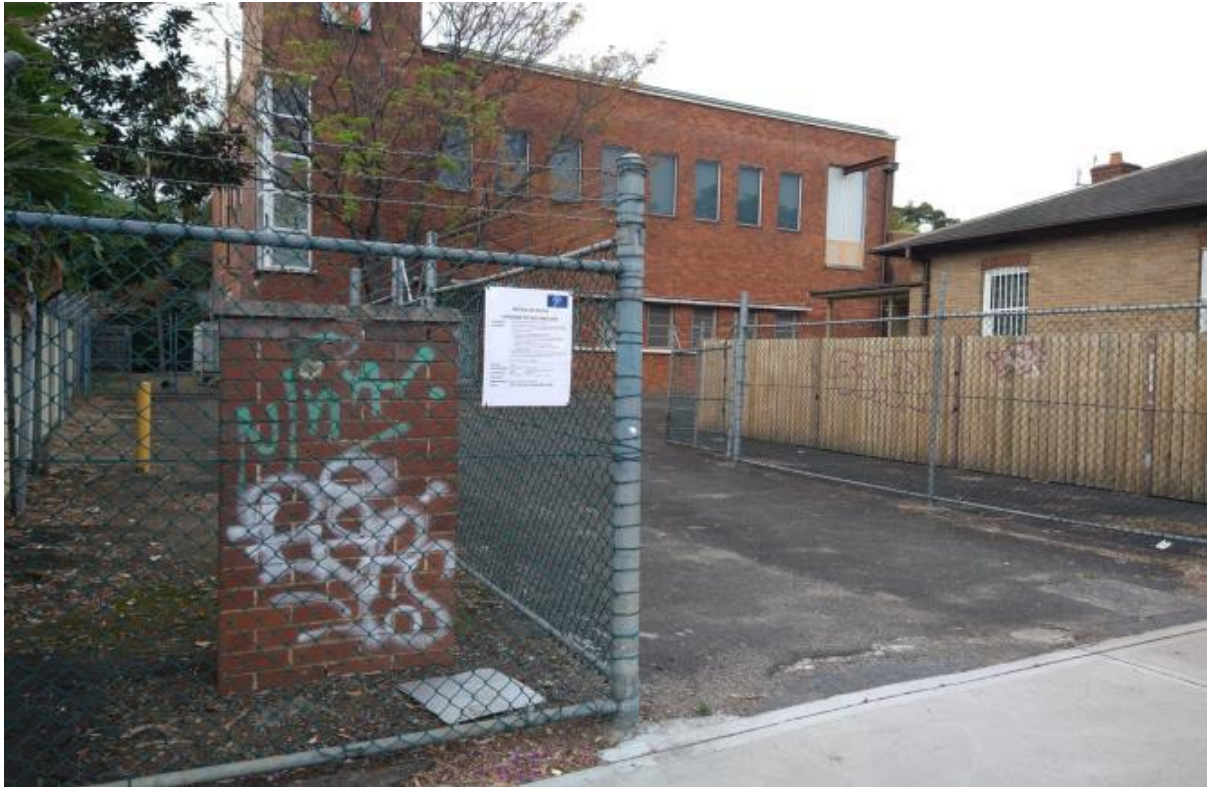
Photo 1 Telstra Cremorne exchange showing graffiti – 10 July 2022
