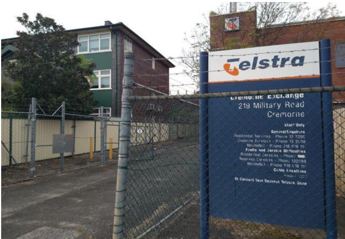
Photo 2 Telstra Cremorne exchange showing unkept appearance- 10 July 2022
