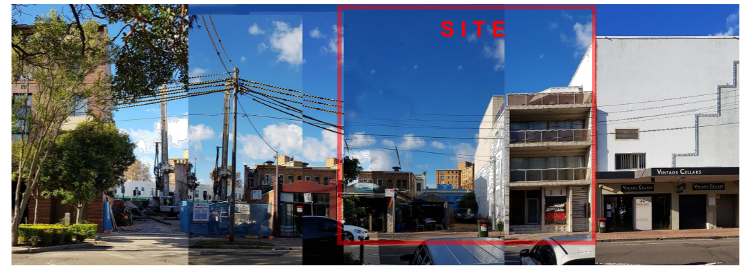
STREET VIEW ALONG PARRAWEEN STREET
