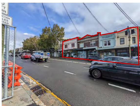
FIGURE 5: Heritage-listed “Higgins Buildings” terraces to the north of the site.
