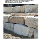
17. REUSED SANDSTONE RETAINING WALLS
