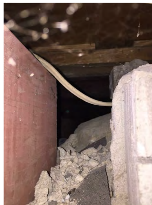
4 - VISUAL ACCESS PAST BEAM IN BASEMENT TO UNDER GROUND FLOOR
