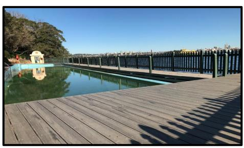
The fencing posts, rails and pickets have been replaced with a HDPE product called "Plastiwood". This product is specifically designed to replicate the original timber fence. It will be able to withstand the harsh marine environment at this location and reduce the overall maintenance requirements compared to the original timber fence.
