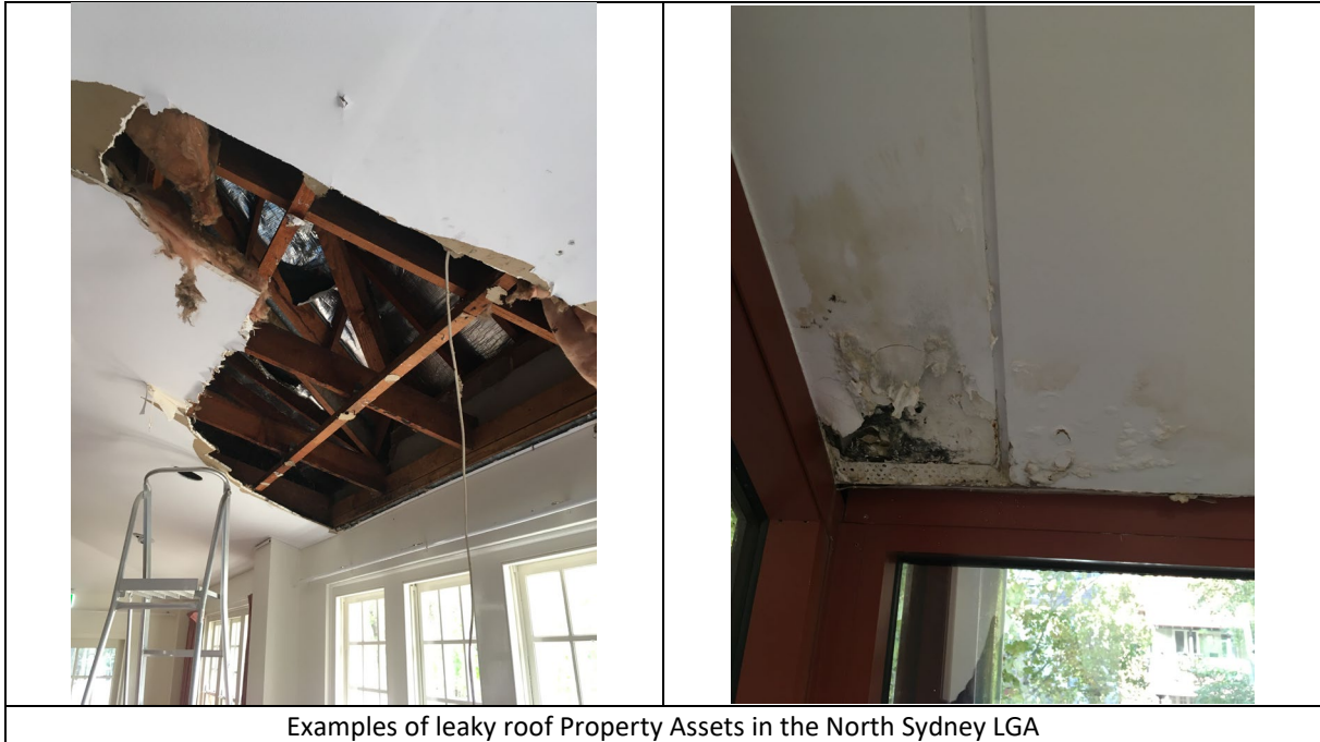
Examples of leaky roof Property Assets in the North Sydney LGA
