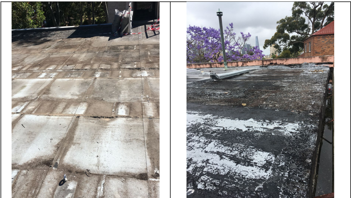
Examples of failed waterproofing on flat roofs
