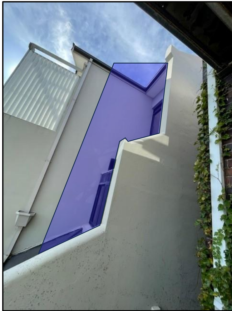
Figure 1: Existing southern elevation of subject dwelling with portion of new southern wall (shaded in blue) that will be close to the boundary and behind the current parapet wall
