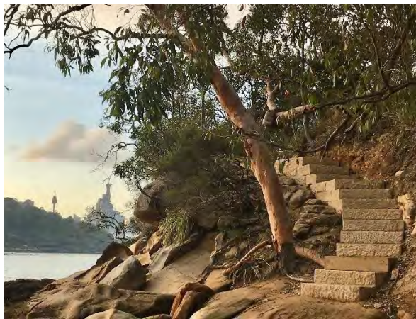
New sandstone stairs to the foreshore
