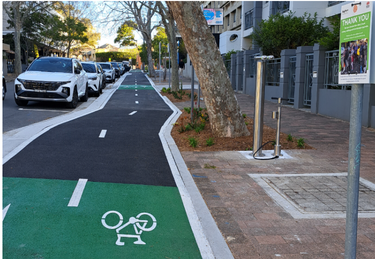
Image 2. Bike pump intersection Ridge Street and West Street
