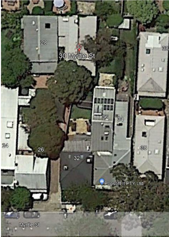
AERIAL PHOTO SHOWING LARGE TREE BETWEEN SUBJECT PROPERTY AND NO. 12 MYRTLE ST.
