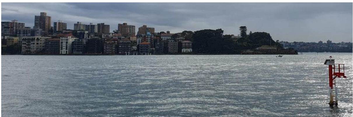
Figure 26: From the Opera House, and in a brighter light, individual buildings become apparent. Toward the centre of the image, the subject building can be identified by the blue lift structure on the roof. Although a dark photo, the colours of the existing building blend in, and the contrasting effect of white balconies and windows is clear. The prominence of the off-white building on the shore and left of the subject building, is evident. As discussed, if all buildings visible in this image were of similar white to pale grey hues, they would collectively compete, and not contrast with, the Opera House.
