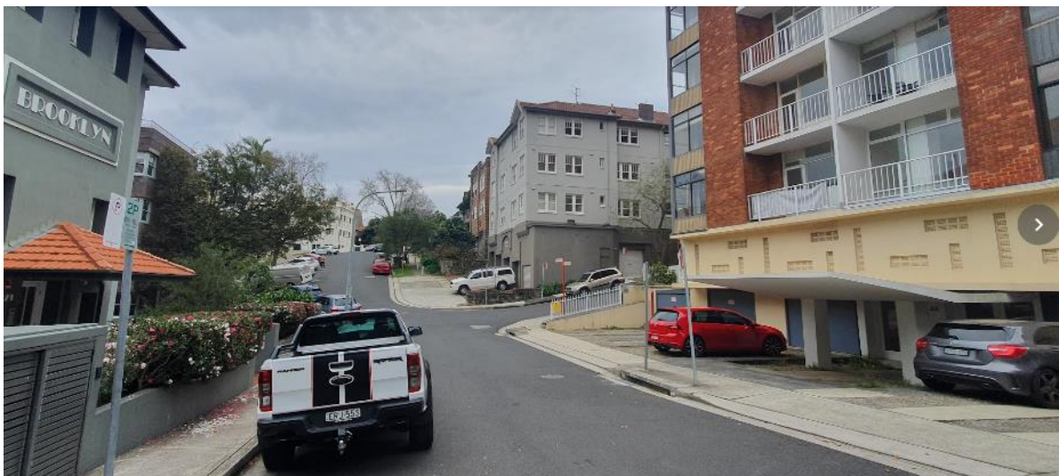
Figure 7: View of the subject building to the right, looking westwards up Waruda Street, the steepness of Beulah Street is indicated and reflected in the tall sublevel of the building in the centre of the image, to the left of the subject building.
