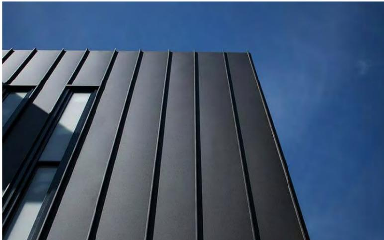
Standing seam metal cladding to stairwell
