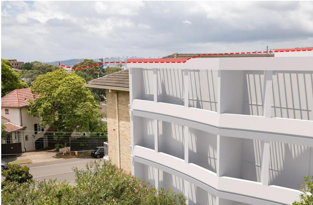
Figure 35 – Revised view impact analysis diagram as viewed from Unit 12 No. 100 Ben Boyd Road. New plant enclosure coloured in red. Red dashed line is 12m height of building development standard line, Gyde Section 4.56 Planning Statement
