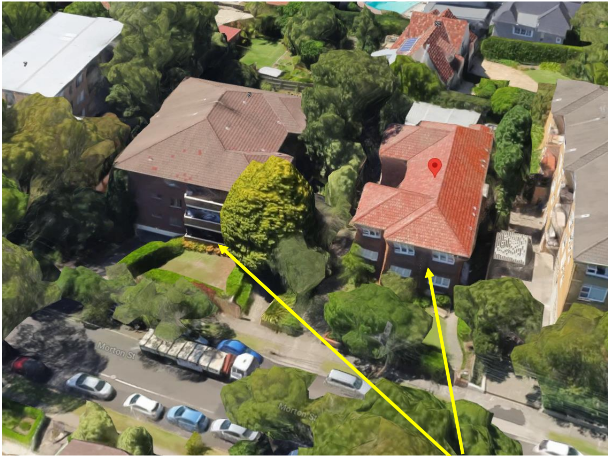
Figure 4. View from the southwest of the subject site and surrounds
