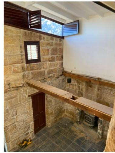
Figure 116.0, Former kitchen space with floor temporarily removed
