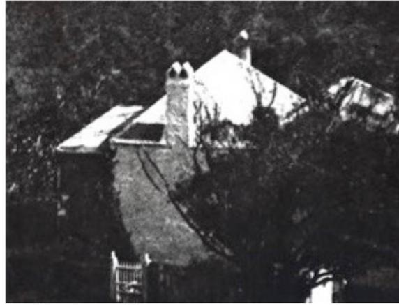
Figure 114.0, Detail of 1875 Holtermann photo showing chimney capping to be reconstructed.
