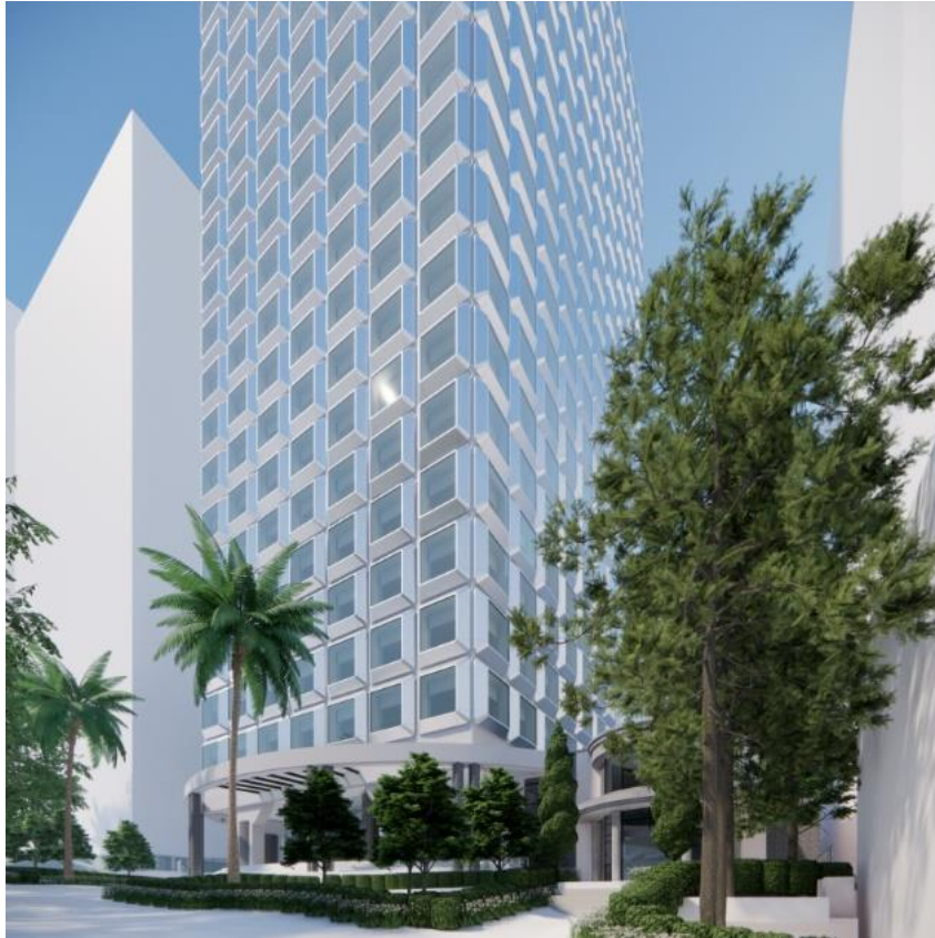
Figure 3: Render prepared by Sissons Architects of the previously proposed works to 201 Miller Street North Sydney with the façade finished in the white powder-coated finish.
