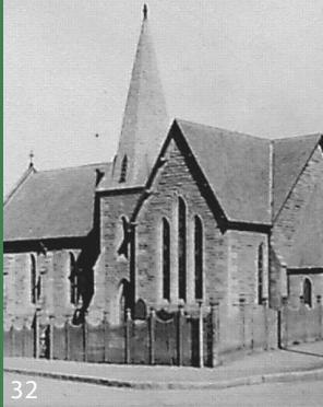
MISSING CORNERS Cnr Pacific Highway Blue and Walker Streets North Sydney
