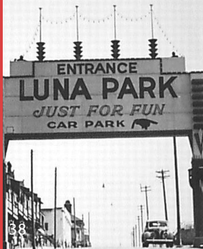
LUNA PARK GATEWAY Alfred Street Bradfield Park South Milsons Point
