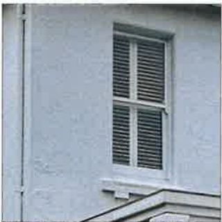
W - Proposed Windows - to original house - timber framed to match existing
