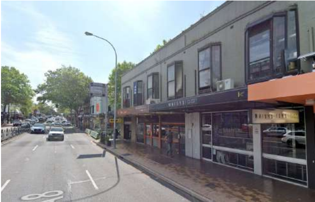
Figure 19 Two storey shops at the west
