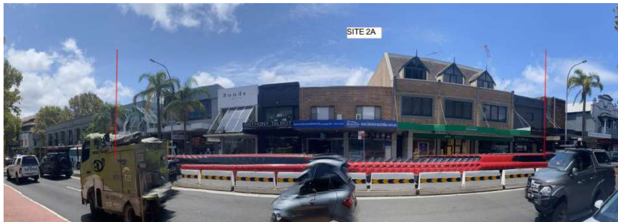
FIGURE 12: Site 2A viewed from Military Road
