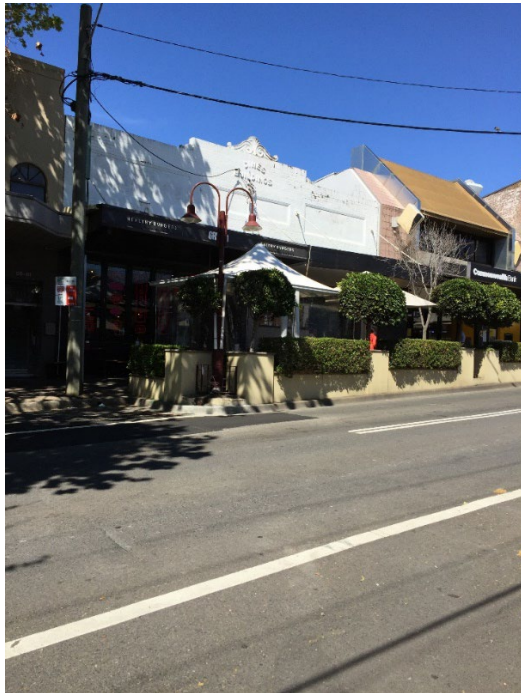
Figure 16 Building stock character
