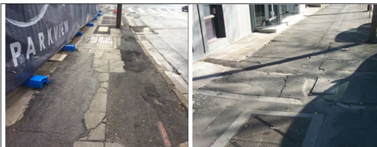
Utility services restorations/reinstallments
