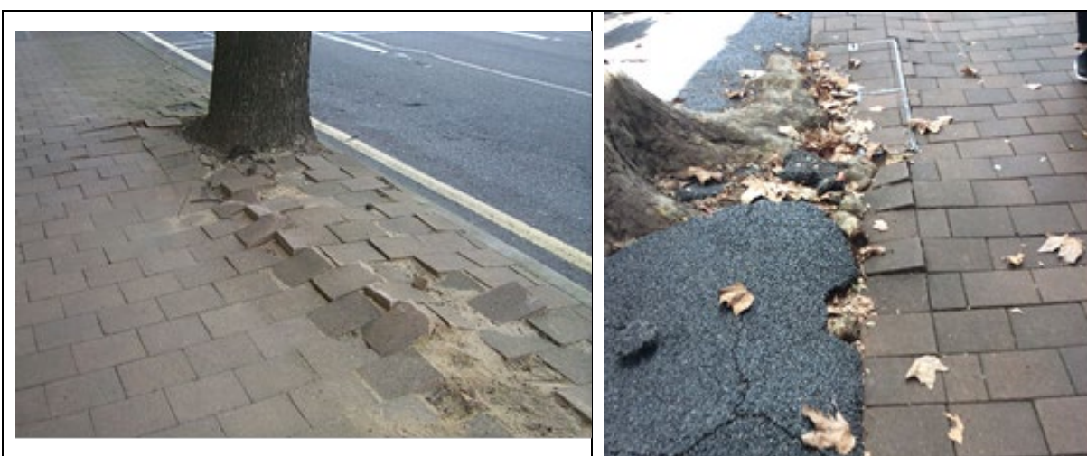
Tree root affected pavers and tree site infill
