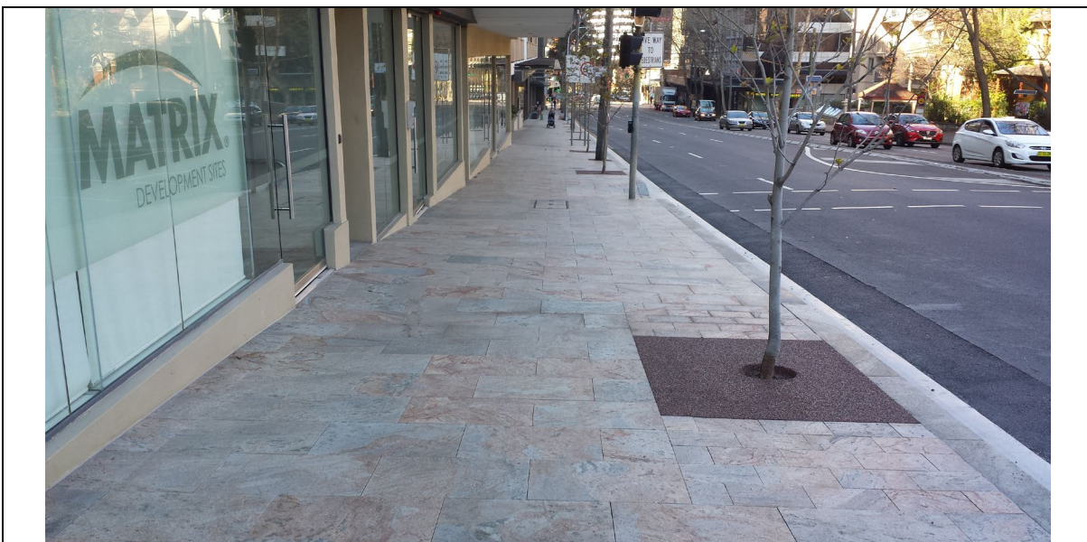
Pacific Highway, North Sydney – Granite
