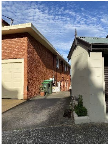
Figure 20. View 1a Waiwera &amp; existing wall 49 East Crescent St
