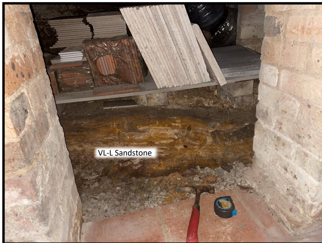
Plate 3 – Southern portion of basement
