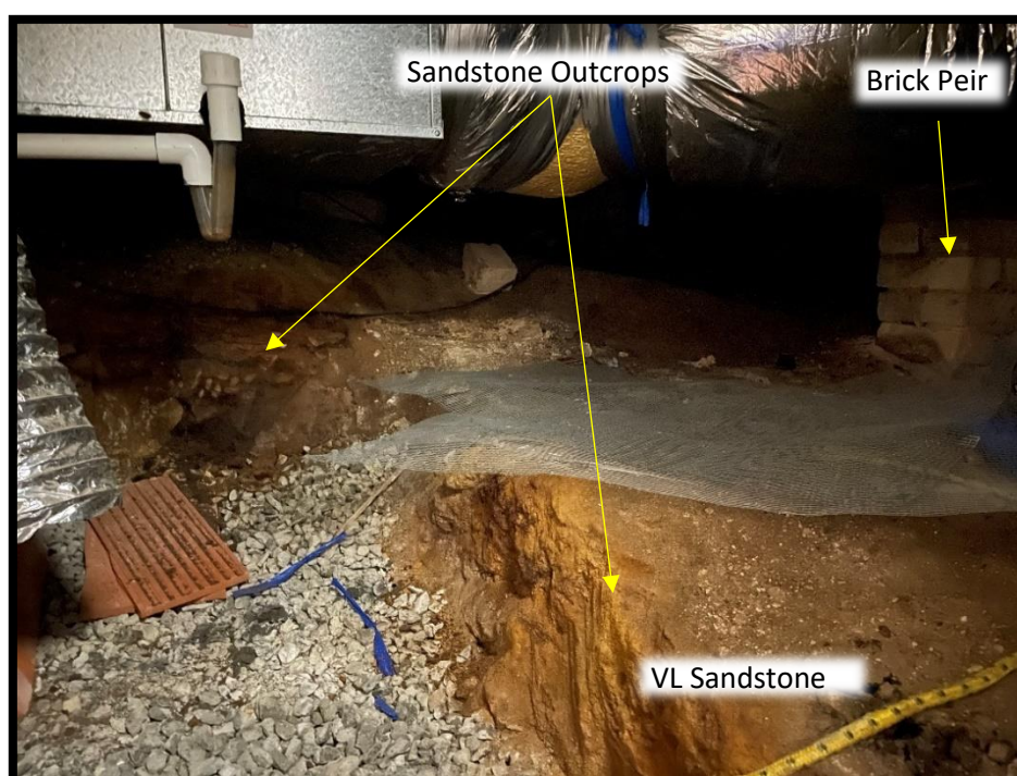
Plate 1 – Centrally within basement
