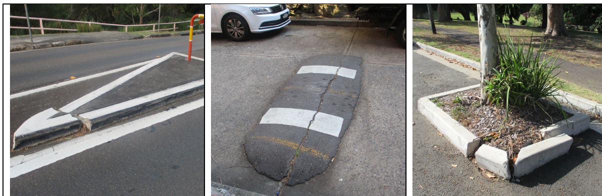
Examples of failed and failing Traffic Facilities in the North Sydney LGA
