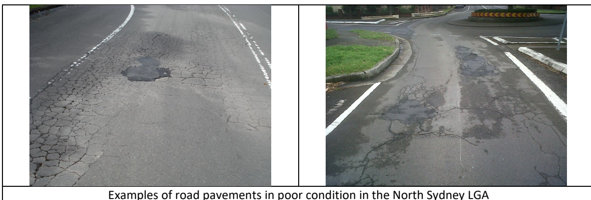
Examples of road pavements in poor condition in the North Sydney LGA
