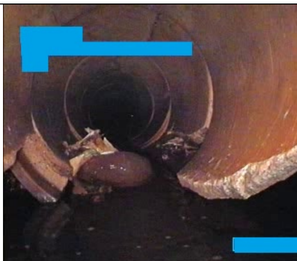
Stormwater Pipes in very poor condition – collapsed
