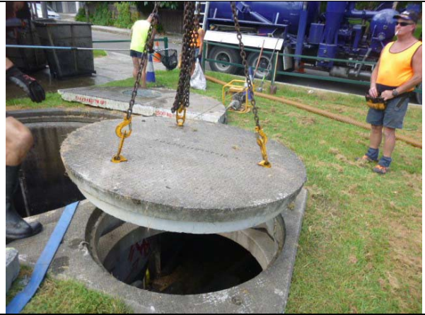
Lids are too heavy - The wood is starting to chip; they should be replaced. Lifting points rusted or broken off
