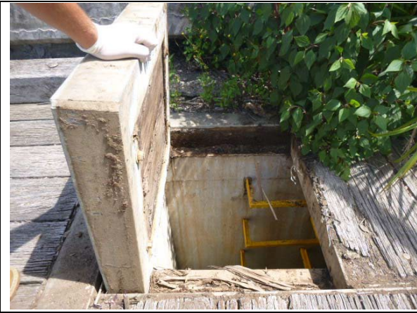
Lids are too heavy - The wood is starting to chip; they should be replaced. Lifting points rusted or broken off
