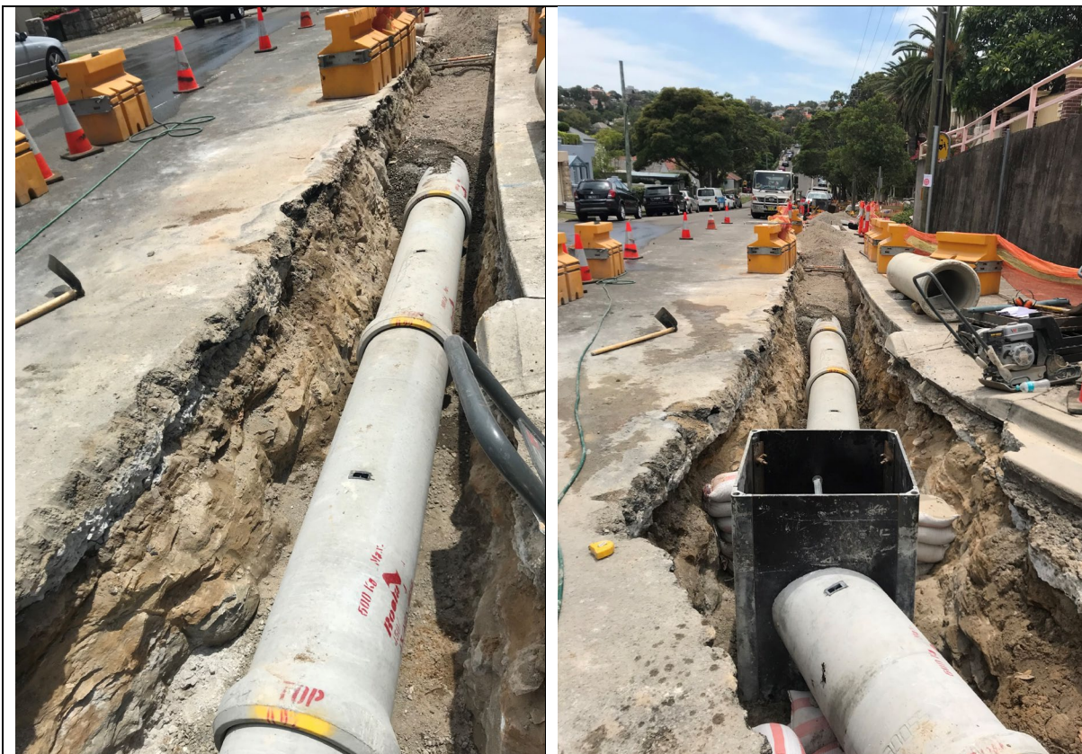
Pit and Pipe replacement at Milson Road, Cremorne Point.
