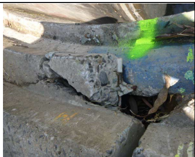
Corrosion and structural damage to GPT manhole covers
