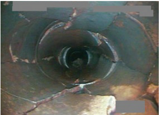
Pipe in very poor condition
