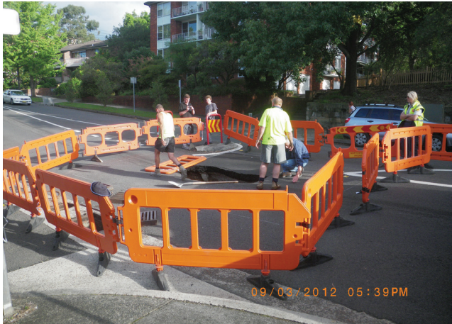
Sink hole in road near defective pipe
