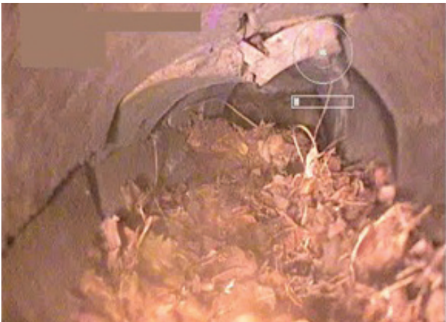
Pipe in very poor condition
