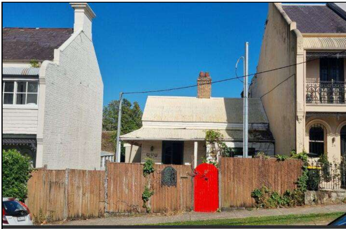
Figure 3: No 22 Chuter Street with terrace houses at No 20 to the left and No 24 to the right
