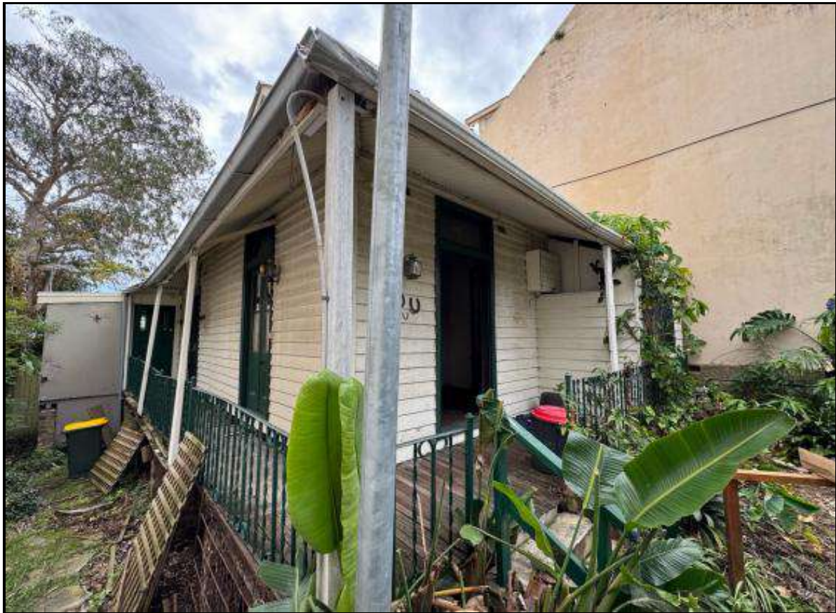
Figure 4: Front façade and southern elevation of existing dwelling with external wall of No 24 to the right
