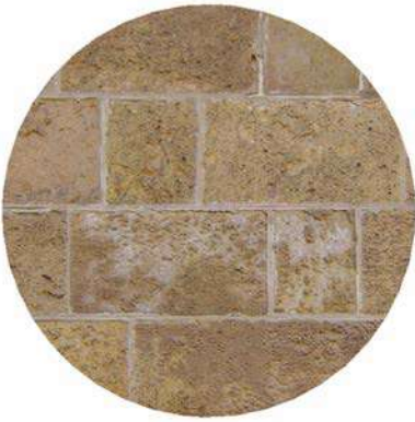
ST: SANDSTONE WALL RUSTICATED FINISH
