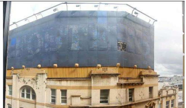
Existing situation – view from adjoining hotel
