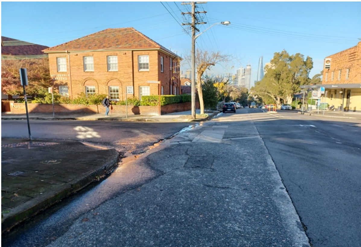
Photo 2. The existing site – 21/06/22
