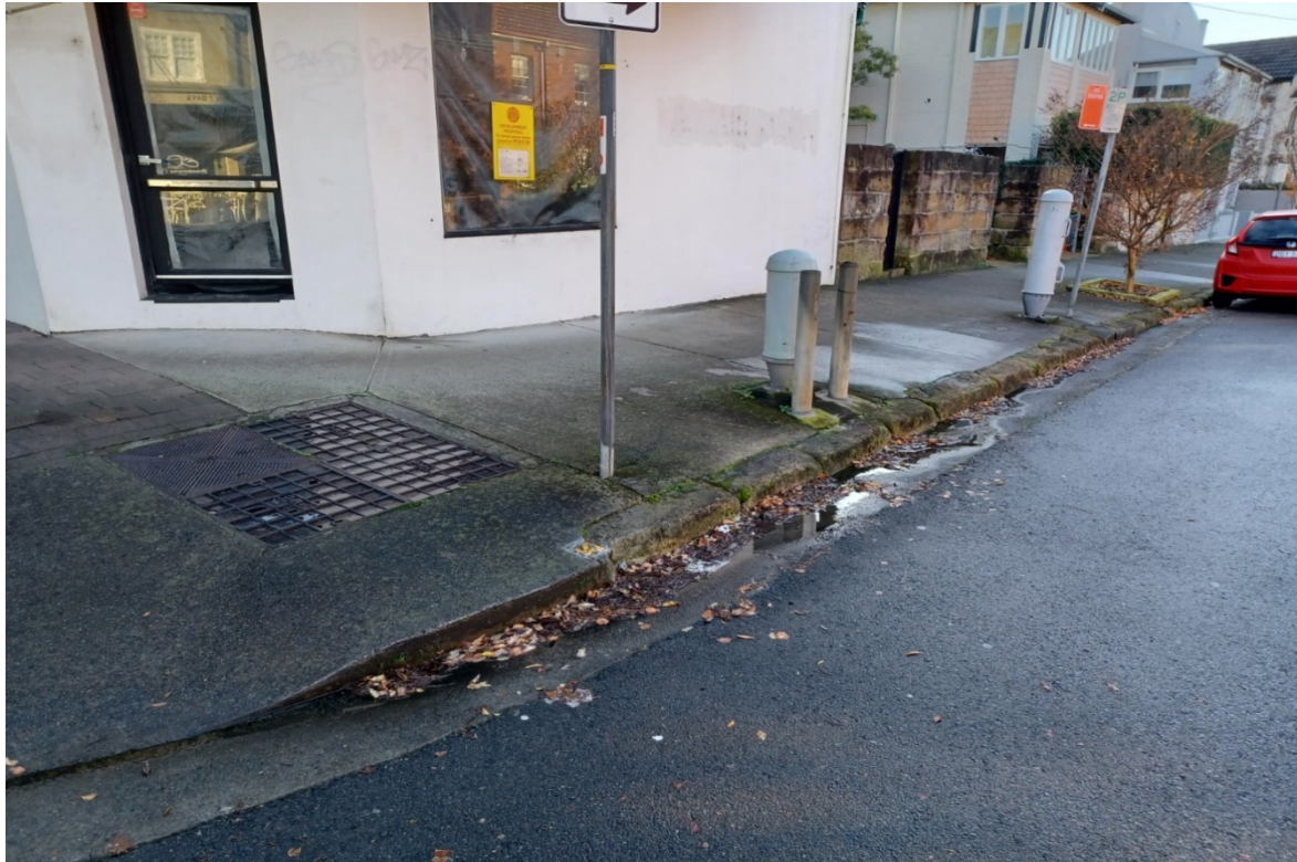
Photo 5. The existing site – 21/06/22
