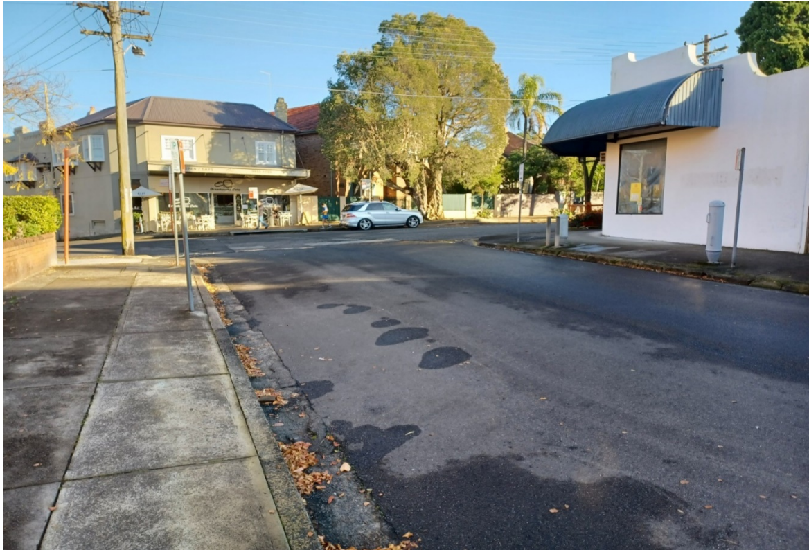
Photo 3. The existing site – 21/06/22
