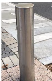
Stainless steel bollards to North Sydney Council standards
