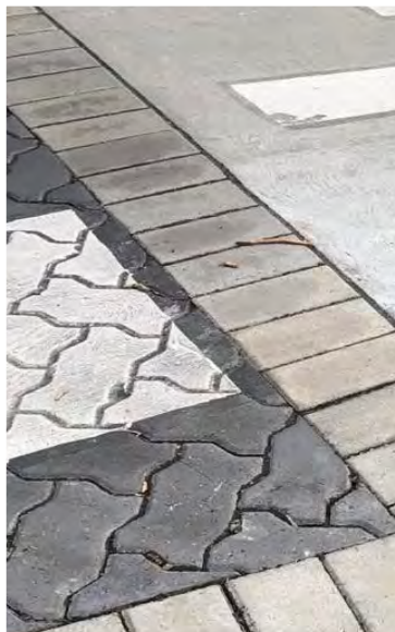
Interlocking concrete pavers with soldier course frame
