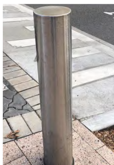
Stainless steel bollards to North Sydney Council standards
