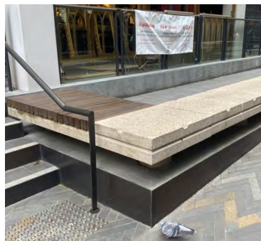
Precast feature seating edge takes up level change
