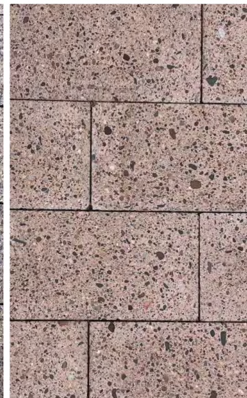
Precast concrete unit paver 2
