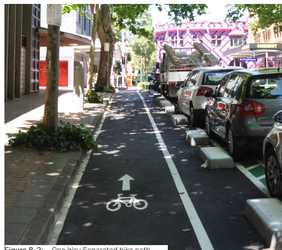
Figure 8-2: One Way Separated bike path One Way Separated Bike Path
