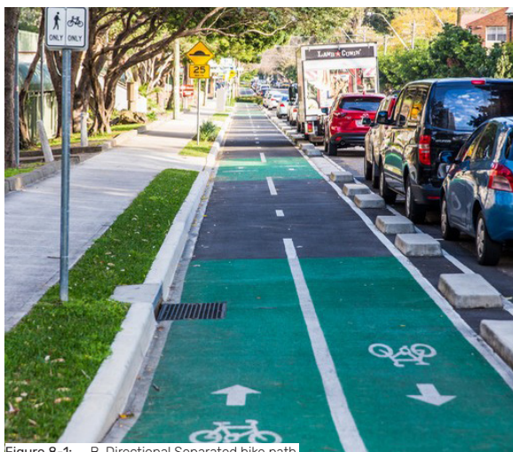
Figure 8-1: B-Directional Separated bike path Bi-Directional Separated Bike Path
