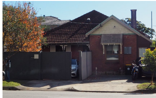
Figure 3. 21: Nos. 70 &amp; 72 Parraween Street, the most intact of the semi-attached pairs of cottages.
