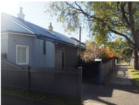
Figure 3. 17: Nos. 52 to 56 Parraween Street, a row of attached workers cottages dating from c.1889.
