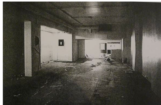
Figure 2. 54: Western-most shop to the ground floor. Source: Rod Howard Heritage Conservation, March 1998
