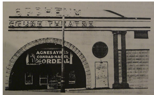
Figure 2. 24: View of the exterior of the first North Sydney Orpheum Picture Theatre, showing the entrance arch, imitation pillars and iron gates. Source: Clark, John Stephen, “Orpheum Theatre,” Kino: Journal of the Australian Theatre Historical Society 7, No. 3 (March 1989): 7
