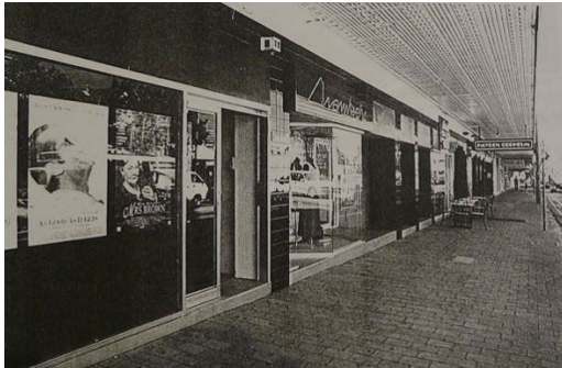
Figure 2. 51: Front facade (Military Road) in 1998. Source: Rod Howard Heritage Conservation, Statement of Heritage Impact, March 1998
