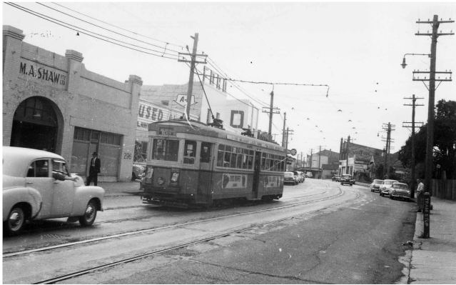
Figure 2. 21: 1950s photograph of Military Road between Winnie and Paling Street. Source: Stanton Library
