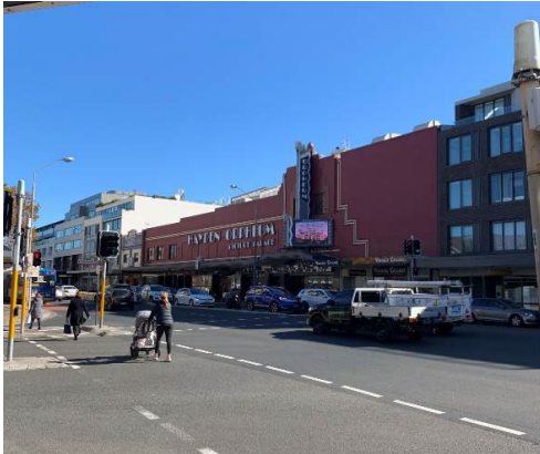
Figure 3. 61: Front façade of the Cinema viewed from Military Road.
