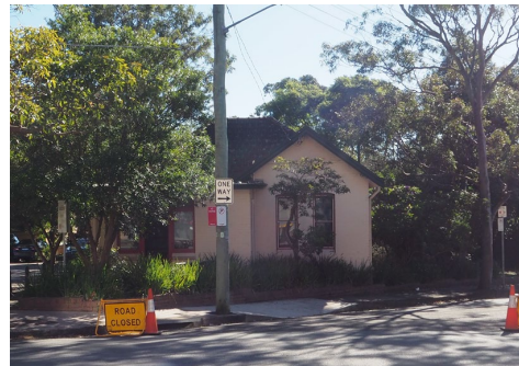
Figure 3. 14: No. 108 Parraween Street, one of the free-standing cottages developed by Helier Harbutt in the early 20 th century and now in use as a family health clinic.
