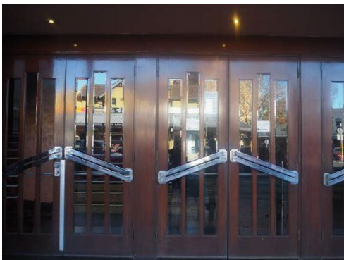
Figure 3. 63: Entry doors to original foyer (possibly original).
