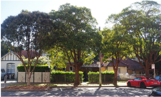
Figure 3. 15: Nos. 82 to 86 Parraween Street, the free-standing cottages constructed by Helier Harbutt.
