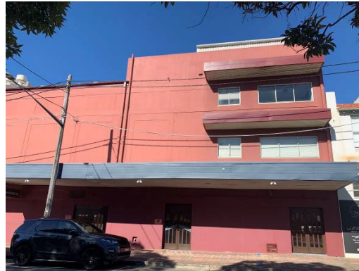
Figure 3. 68: Western side of the rear of the Cinema, showing the original location of the fly tower (converted to offices).
