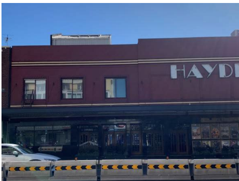
Figure 3. 65: Western side of the Cinema. The structure of the fly tower is visible over the parapet.
