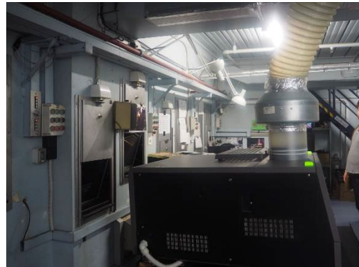
Figure 3. 80: Projection room to main auditorium
