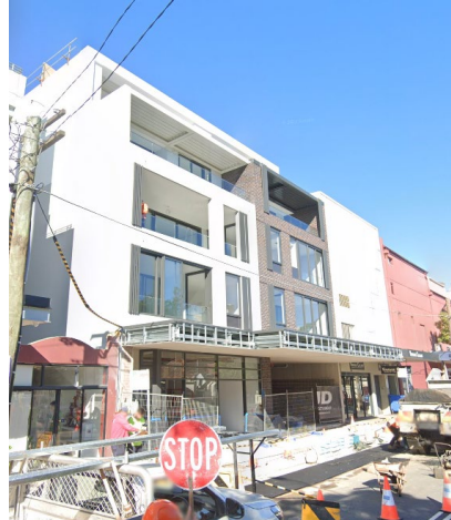
Figure 3. 96: The rear elevations of No. 390-394 Military Road, as seen from Parraween Street.
