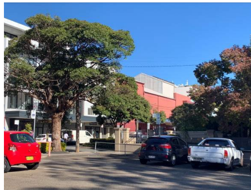
Figure 3. 60: View towards the rear elevation of the Cinema from Parraween Street carpark.
