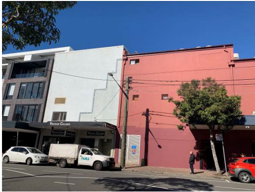
Figure 3. 67: Eastern side of the rear of the Cinema. The adjoining building painted white now forms part of the complex.
