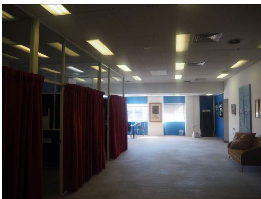
Figure 3. 88: Second floor offices, in location of fly tower
