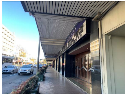
Figure 3. 64: Awning over original entry foyer, looking west.
