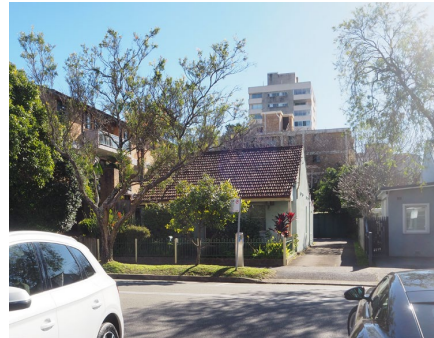
Figure 3. 16: No. 50 Parraween Street, a free-standing cottage that survives as the oldest building on this portion of Parraween Street.
