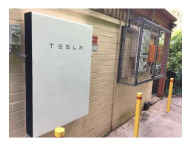
The battery system has been sized to maximise on-site consumption of solar electricity, by charging from excess solar generation during the middle of the day and discharging when solar generation is less than the on-site consumption i.e. during peak hours and/or during non-sunlight hours.
