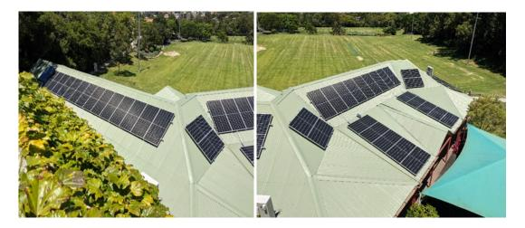
The system comprises a 3-phase SolarEdge Inverter of 17 kW capacity complete with 44 x SolarEdge optimisers and 1 x Tesla Powerwall batteries (1 x 13.5kWh). The Tesla battery
