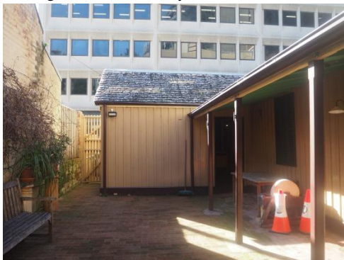
Figure 3.19: Rear yard looking north.
