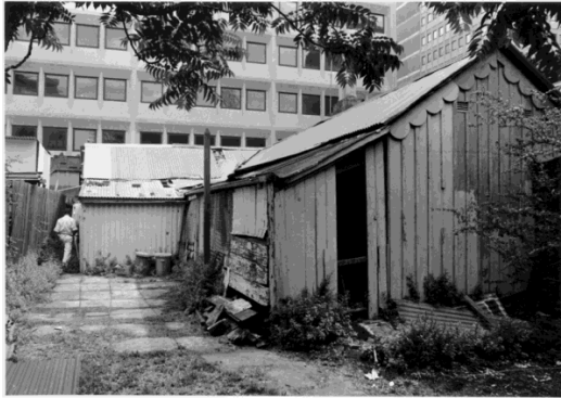
Figure 2. 40: Rear elevation of Don Bank prior to restoration works in c.1975. Courtesy: G. Britton
