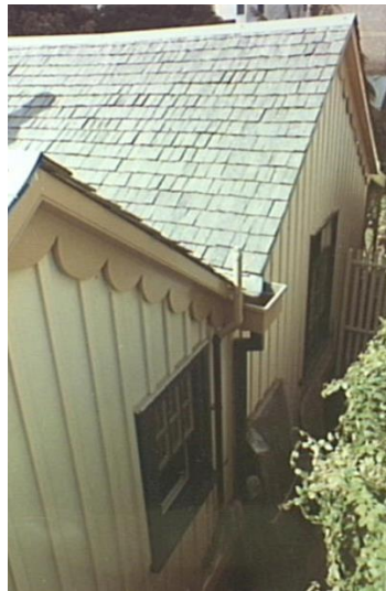
Figure 2. 49: The restored roofing of shingles. Source: Stanton Library (CPF 324)
