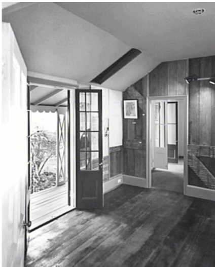
Figure 2. 48: The interior of Don Bank after completion of restoration works in 1981. Source: Stanton Library (PF 2925)
