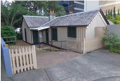
Figure 3. 26: North and west elevations of kitchen wing attached to rear elevation of main body of the cottage.
