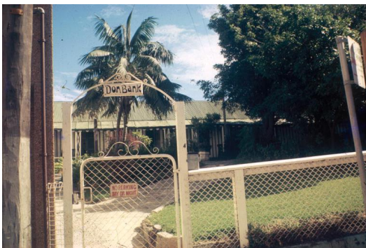
Figure 2. 50: Don Bank after completion of restoration works. Source: Stanton Library
