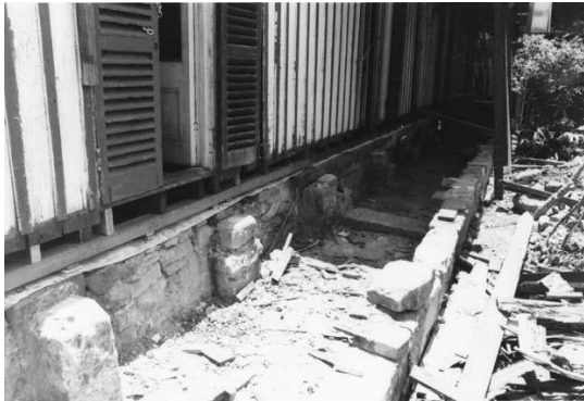
Figure 3. 68: Front verandah during conversion, c1979
