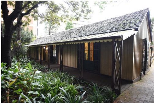
Figure 3. 24: Front (east) elevation
