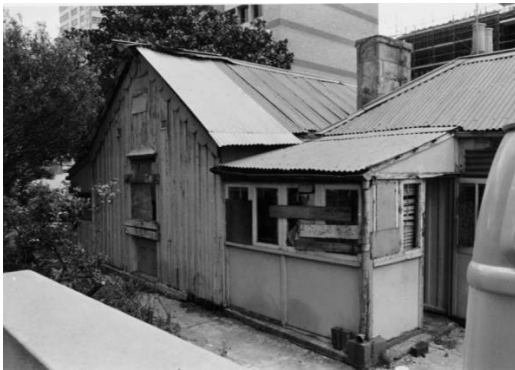
Figure 2. 38: View of the north elevation of the house and entry porch leading into the rear kitchen wing of Don Bank prior to restoration. Source: Stanton Library
