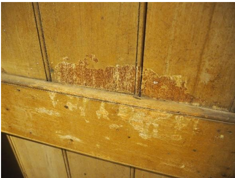
Figure 3. 70: Rail and boards in Space 05 with shiplap joints and a shaped beaded profile.
