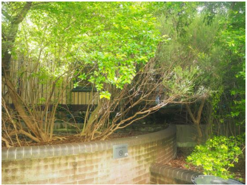
Figure 3. 6: View V4 showing the south elevation of Don Bank as seen through landscaping from the adjacent park to the south.
