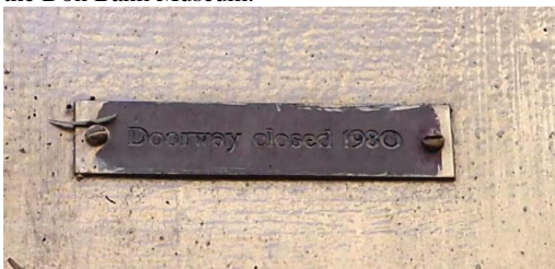
Figure 3. 62: A small plaque indicating the location of an earlier doorway.
