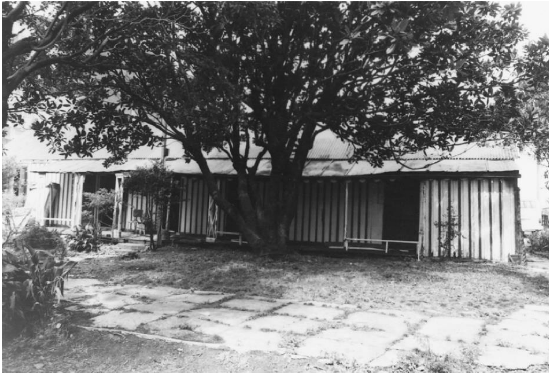
Figure 2. 37: Front elevation of Don Bank prior to restoration works in c.1975. Courtesy: G. Britton
