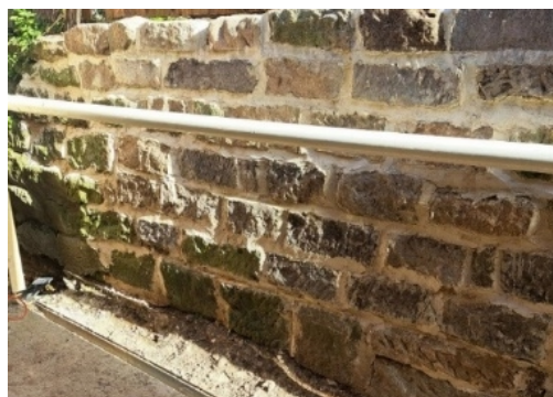
Figure 1: Re-constructed wall once drainage works were complete
