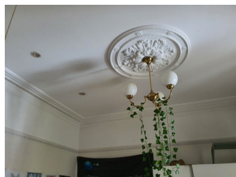
Figure 2. 152: Ceiling to living room with ceiling rose, later down lights, original cornice and picture rail.
