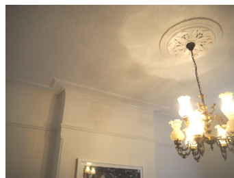
Figure 2. 72: Detail of original cornice, picture rail and ceiling rose to living room.
