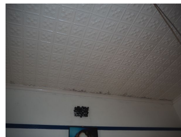
Figure 2. 83: Pressed metal ceiling to front bedroom.
