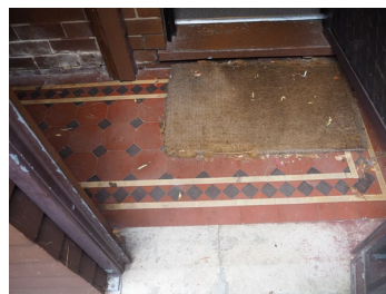
Figure 2. 66: Original encaustic tiles to verandah floor.
