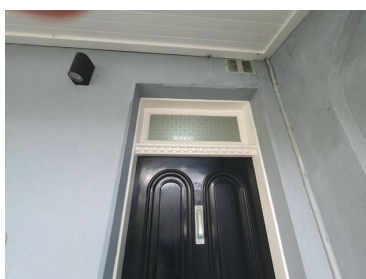
Figure 2. 16: Detail of front door with dentils matching those at No. 50 Parraween Street
