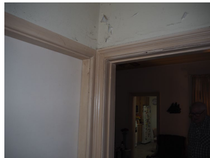
Figure 2. 10: Typical internal architraves.
