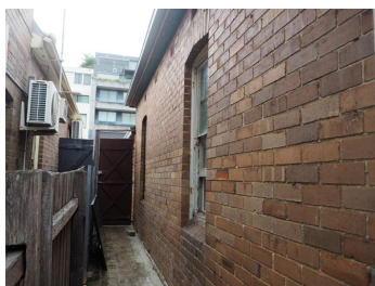
Figure 2. 63:: Side passageway with original windows and boarded eaves.
