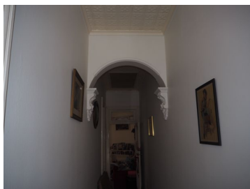
Figure 2. 81: Entry hallway with arched opening and decorative moulded corbels.
