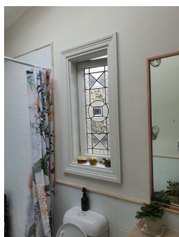
Figure 2. 156: Leadlight glazing to bathroom window.
