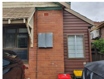
Figure 2. 62: Enclosed side verandah and original timber awning with brackets to front window (replaced with aluminium framed window).
