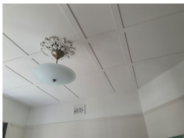
Figure 2. 130: Battered ceiling with ceiling rose and picture rail to master bedroom.
