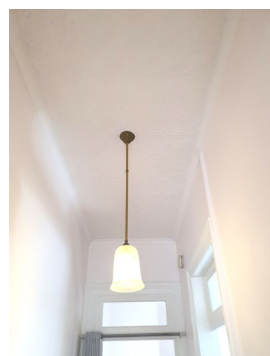
Figure 2. 99: Pressed metal ceiling to hallway.
