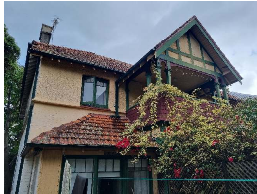
Figure 83. View to first floor and balcony.
