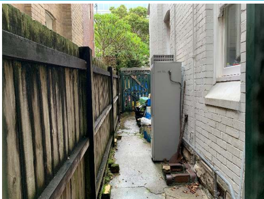
Figure 89. View along western elevation towards Yeo Street.
