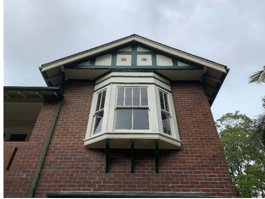
Figure 45. First floor oriel window and gable end.
