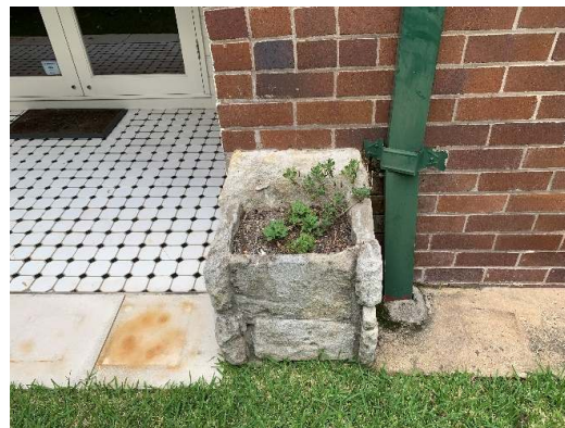
Figure 73. Sandstone planter box in front garden.
