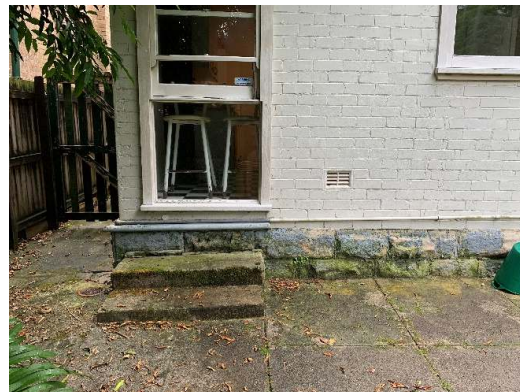
Figure 88. Stairs leading to full-length window.
