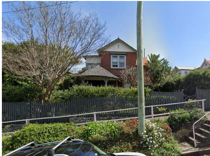
Figure 127. 12 Claude Avenue (Source: Google Streetview 2020).
