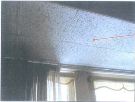
10. Room 4 of ground floor bay window.
