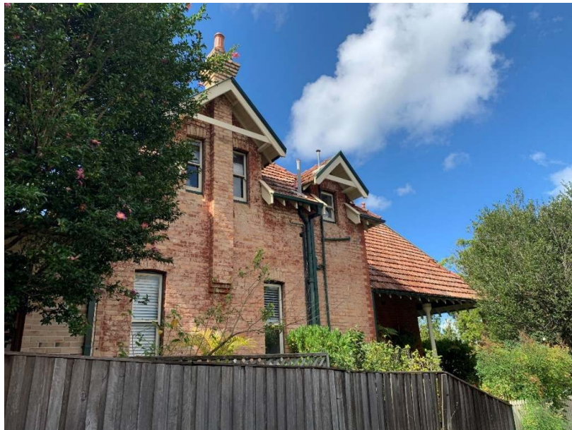
Figure 125. Western elevation of 4 Harrison Street.
