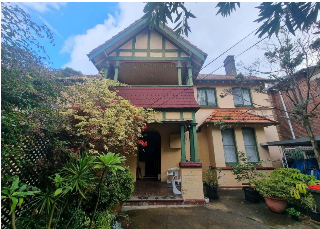
Figure 78. Front façade and entry porch.
