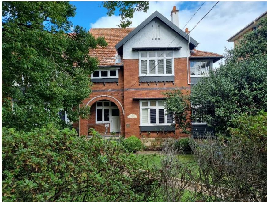
Figure 128. 1 Harrison Street. Addition obscured by vegetation at left.
