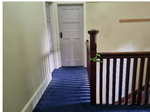
Figure 99. First floor hallway.
