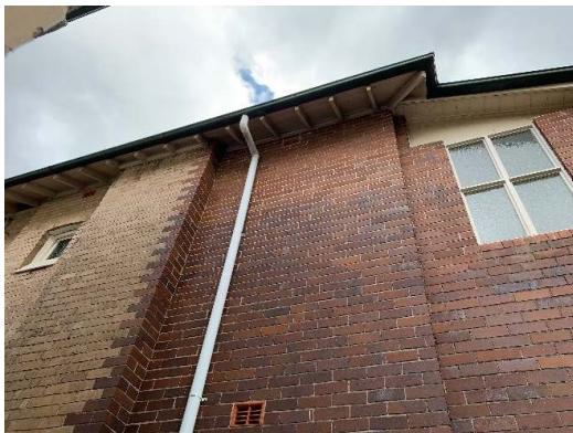
Figure 48. Eastern elevation, balcony window at right.
