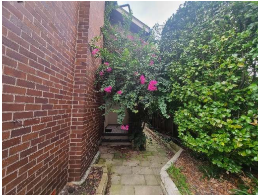
Figure 50. View to entry porch.
