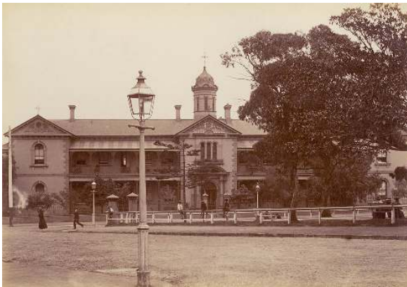
Figure 7 – St Vincent's Hospital after major extensions (on right), including new central turret, designed by Oswald Henry Lewis, photograph dated c1900-1910 (Source: State Library of NSW, PXE 711/211 )
