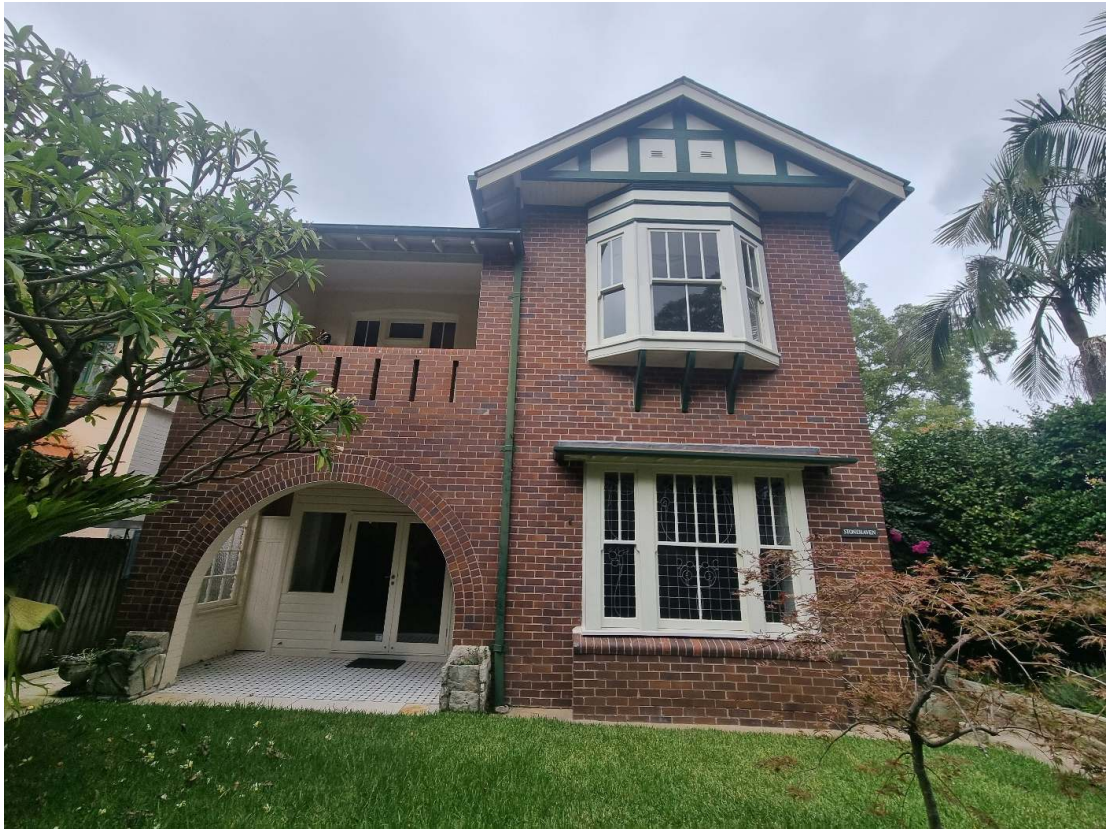
Figure 41. Front façade of 53 Yeo Street.
