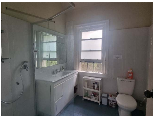
Figure 104. First floor bathroom.
