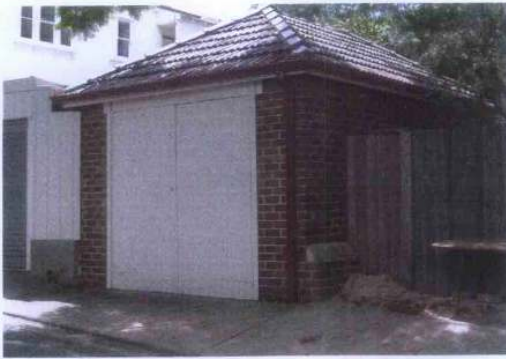
PHOTO 5 Present single garage off Rangers Lane
