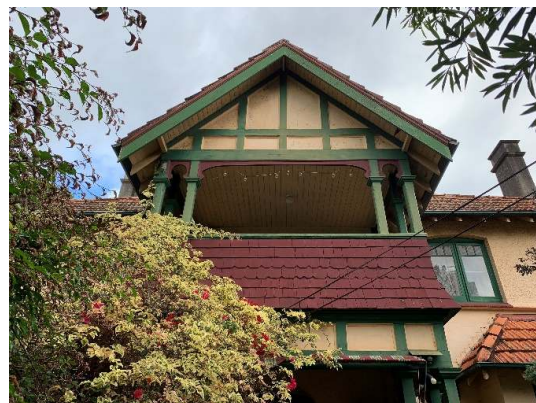
Figure 81. First-floor balcony and singled balustrade.
