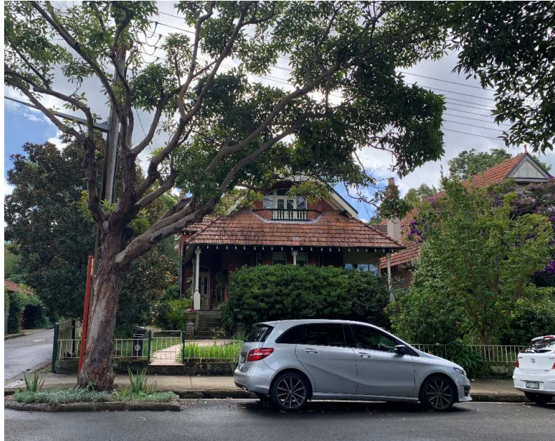
Figure 124. 4 Harrison Street. Rangers Lane at left.
