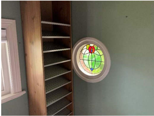
Figure 65. Bulls eye leadlight window in first floor bedroom.
