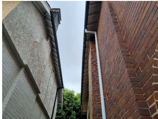
Figure 47. View to upper level of eastern elevation at right.
