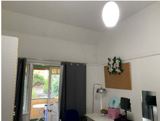
Figure 100. First floor bedroom, door to balcony.
