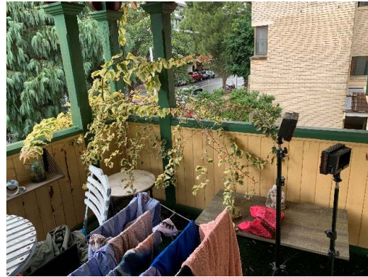
Figure 101. First floor balcony.
