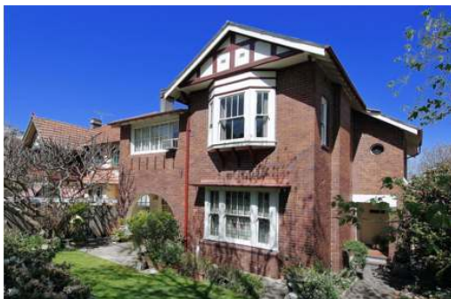
Figure 17 – Photograph showing the Yeo Street elevation with existing balcony window on left and entry on right prior to the 2007 alterations (Source: Luschwitz Cremorne, 53 Yeo Street, Website archived 5 September 2007) 88
