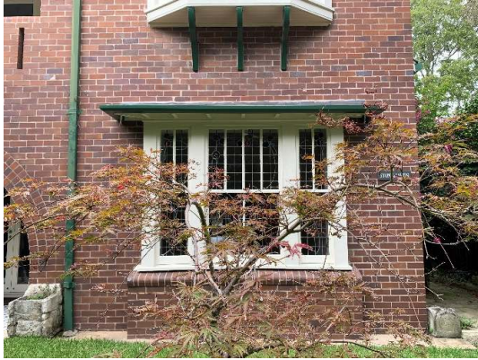
Figure 44. Ground floor window.
