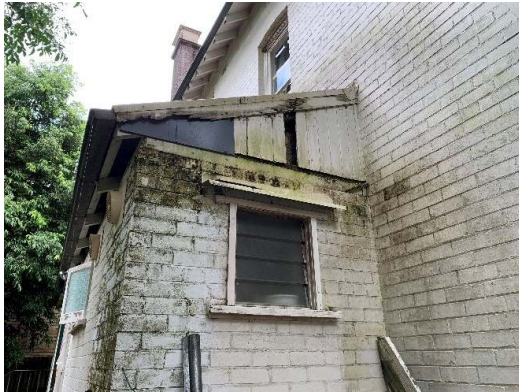
Figure 85. View west to skillion addition.
