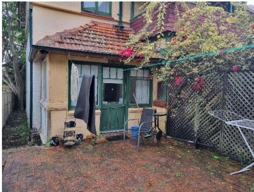
Figure 82. Entrance added in c.1986 alterations.
