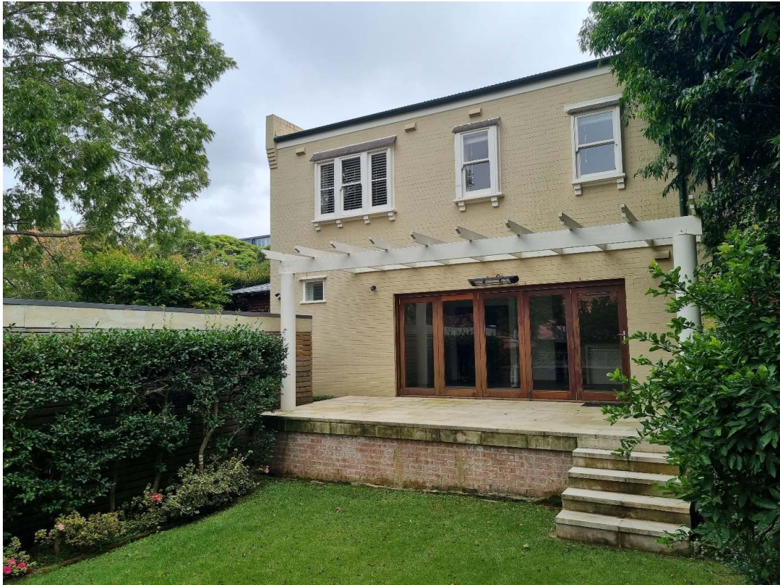
Figure 54. Rear façade of 53 Yeo Street.
