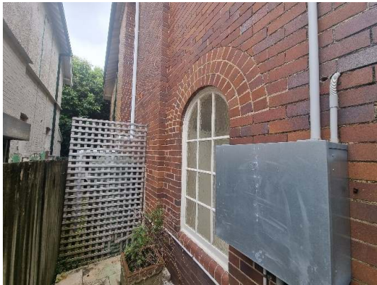
Figure 46. Eastern elevation, showing verandah window.
