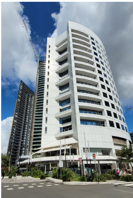
Picture 5 Existing building (looking southwest)
