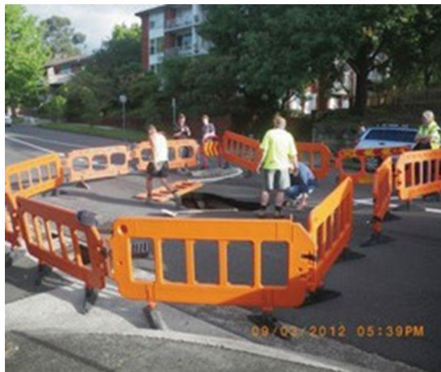
Sink hole in road near defective pipe
