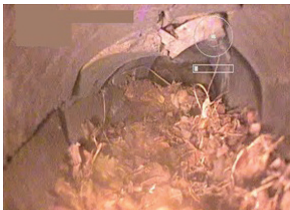
Pipe in very poor condition
