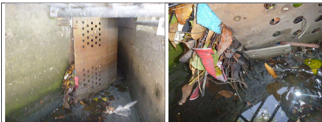
The floatables flap was jammed open due to a broken hinge and pollution trapped in it stopping it closing.
