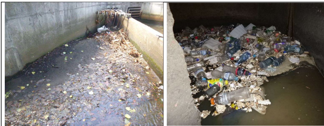
Sediment and trash build up in front of the weir and in pits generally – low capacity.
