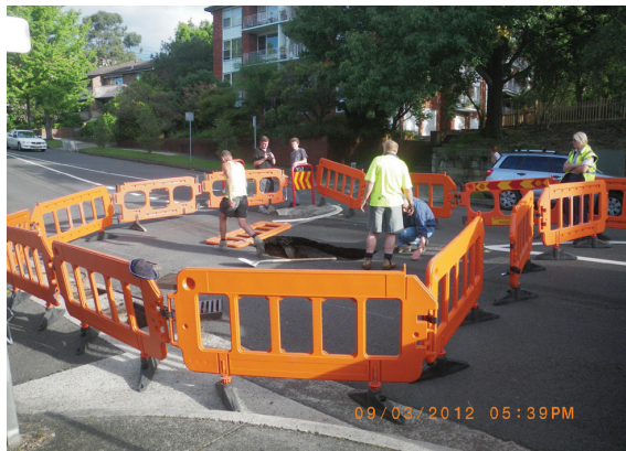
Sink hole in road near defective pipe
