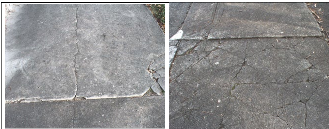
Concrete footpath in poor condition
