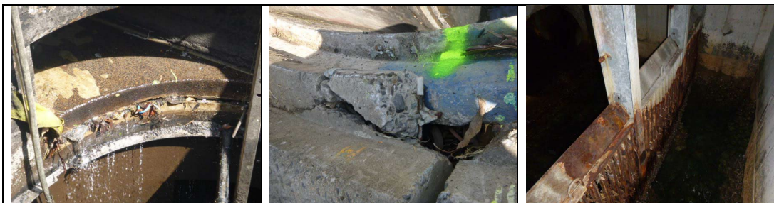
Corrosion and structural damage to GPT manhole covers
