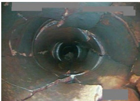
Pipe in very poor condition
