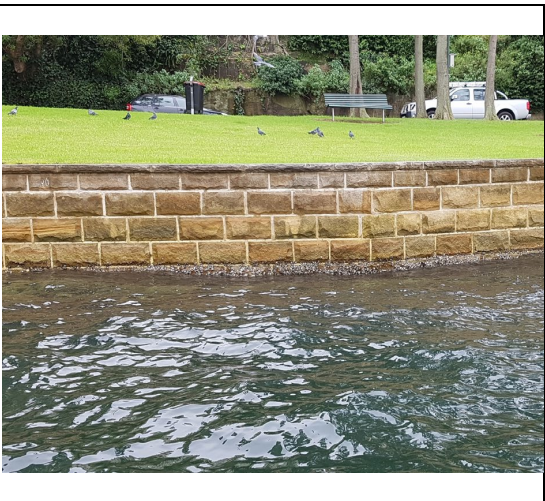
Seawall reconstruction at McMahon's Point -- after
