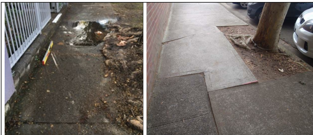
Tree root affected concrete footpath including ponding
