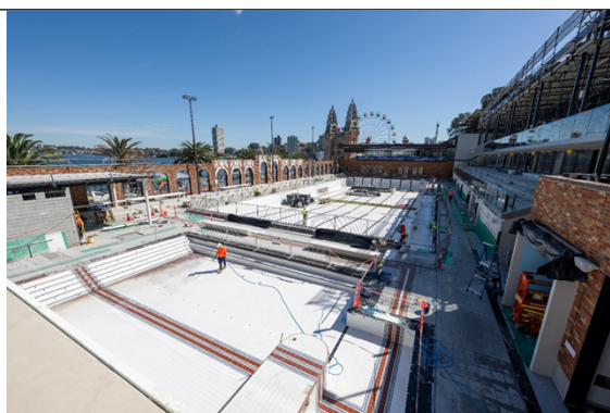
Leisure Pool & Concourse
