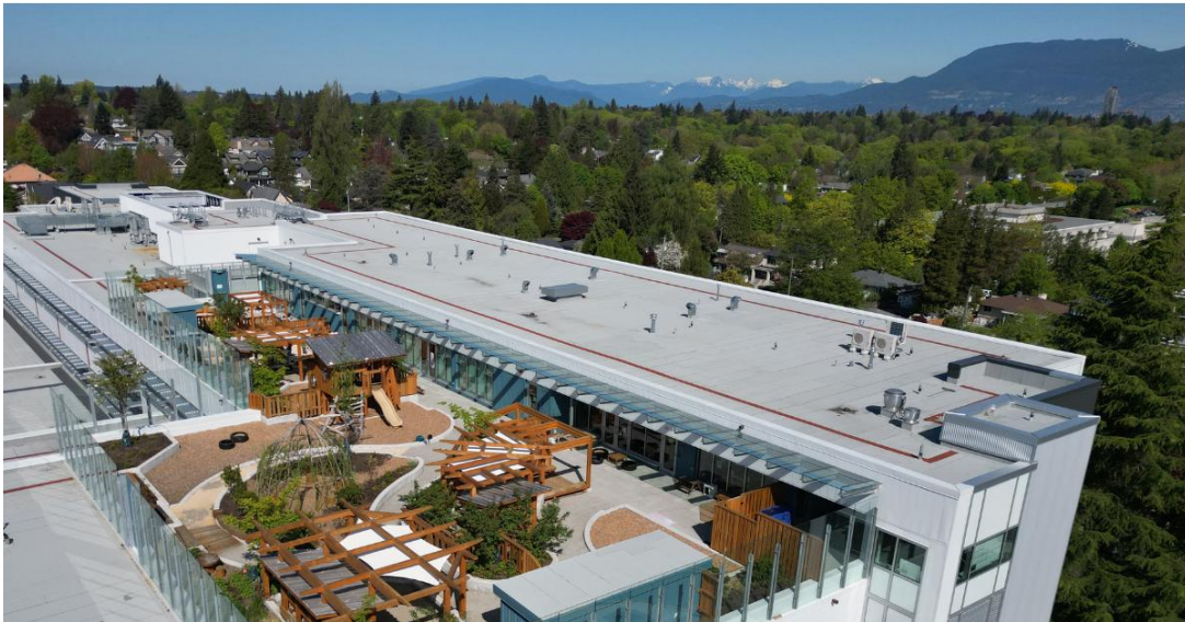
Image: Gastown_ City funded rooftop childcare Vancouver
