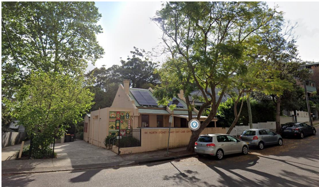
Figure 1_96 Bank Street, North Sydney
