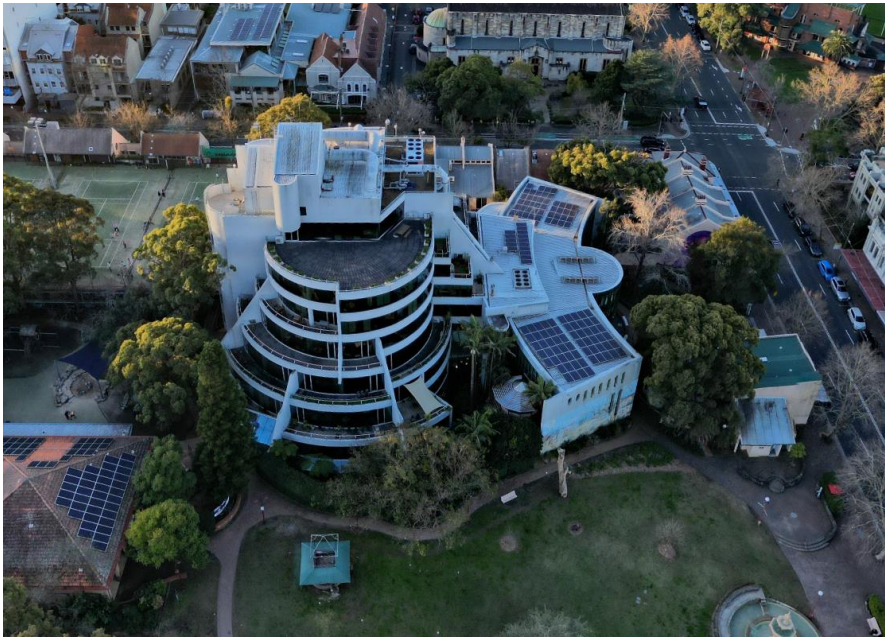
Figure 1_Aerial photograph of the site_Level 6 , 1 James Place, North Sydney
