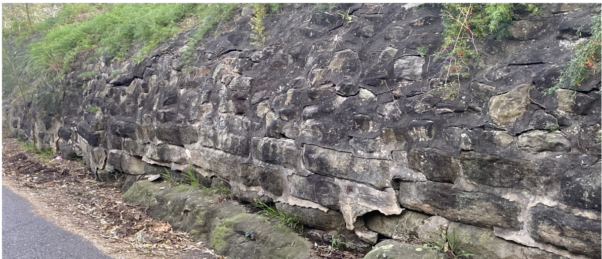
Figure 1: Alfred St Retaining Wall: Deformation (Ch15-35m)
