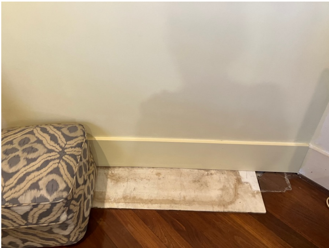
Figure 25: Location of former fireplace in No 29 Bydown Street removed c. November 2025.
