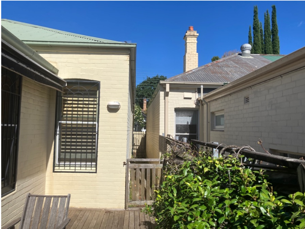
Figure 26: Rear of No. 29 Bydown Street showing adjacent dwelling at No. 31.
