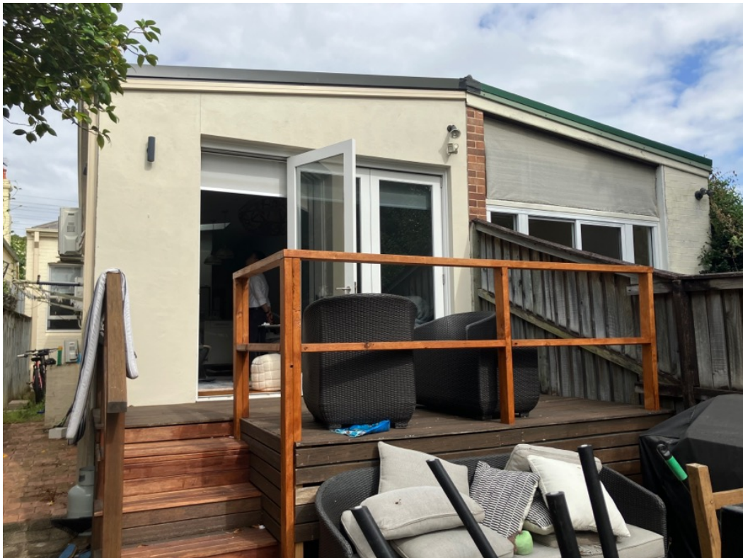
Figure 33: Rear wing of No. 31 Bydown Street, appearing to match the form of its pair at No. 33
