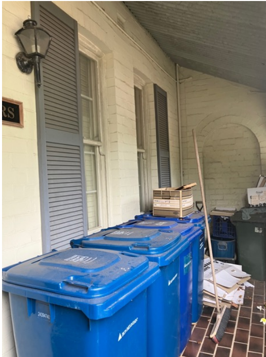
Figure 17: Front entrance verandah of No. 27 Bydown Street showing original form and fenestration with shutters.
