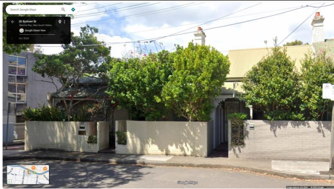
FIGURE 3: 37 & 35 Bydown Street Source – Google Street View 2024 image
