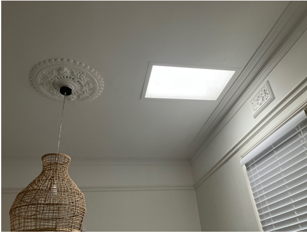
Figure 32:: Front room of No. 31 Bydown Street showing original and likely original features including cornice, picture rail, vent, window, and ceiling rose. Modern skylight.
