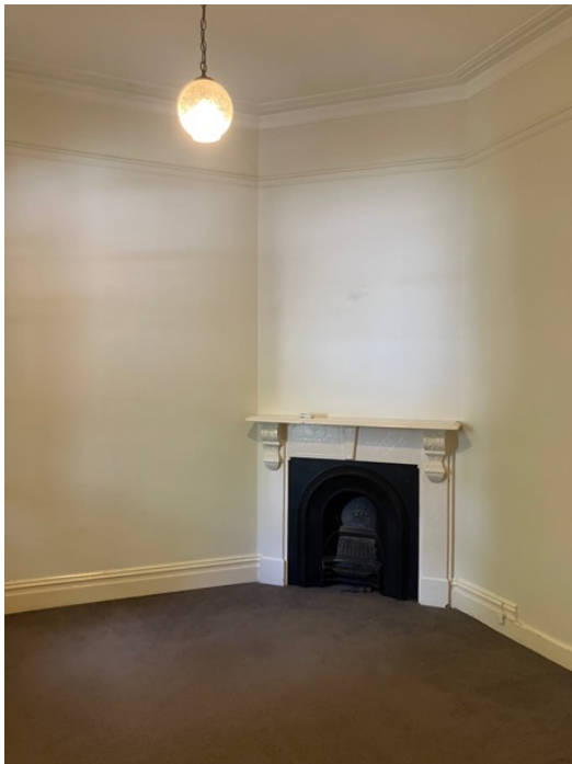
Figure 38: Likely original fireplace and skirting in No. 33 Bydown Street.
