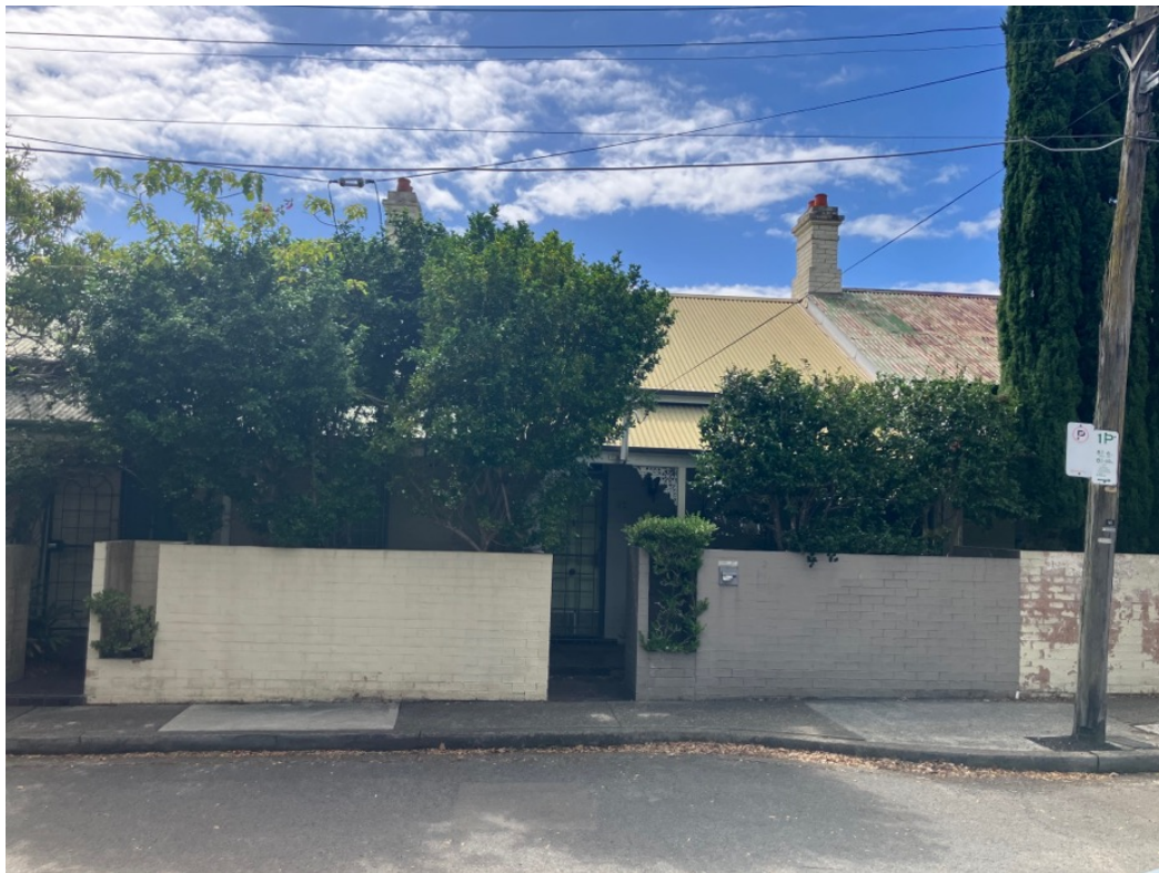
Figure 10: Streetscape presentation of No. 35 Bydown Street, second in the row from the north.
