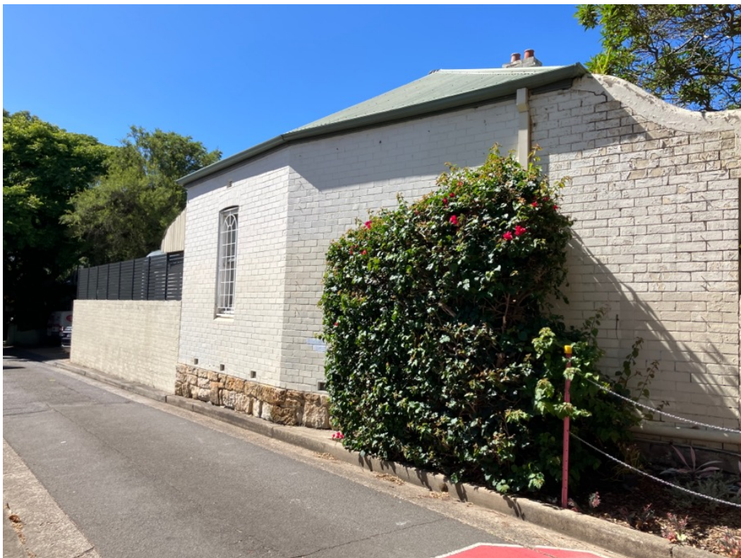
Figure 51: Presentation of No. 37 Bydown Street to Cheal Lane to the north of the cottages.
