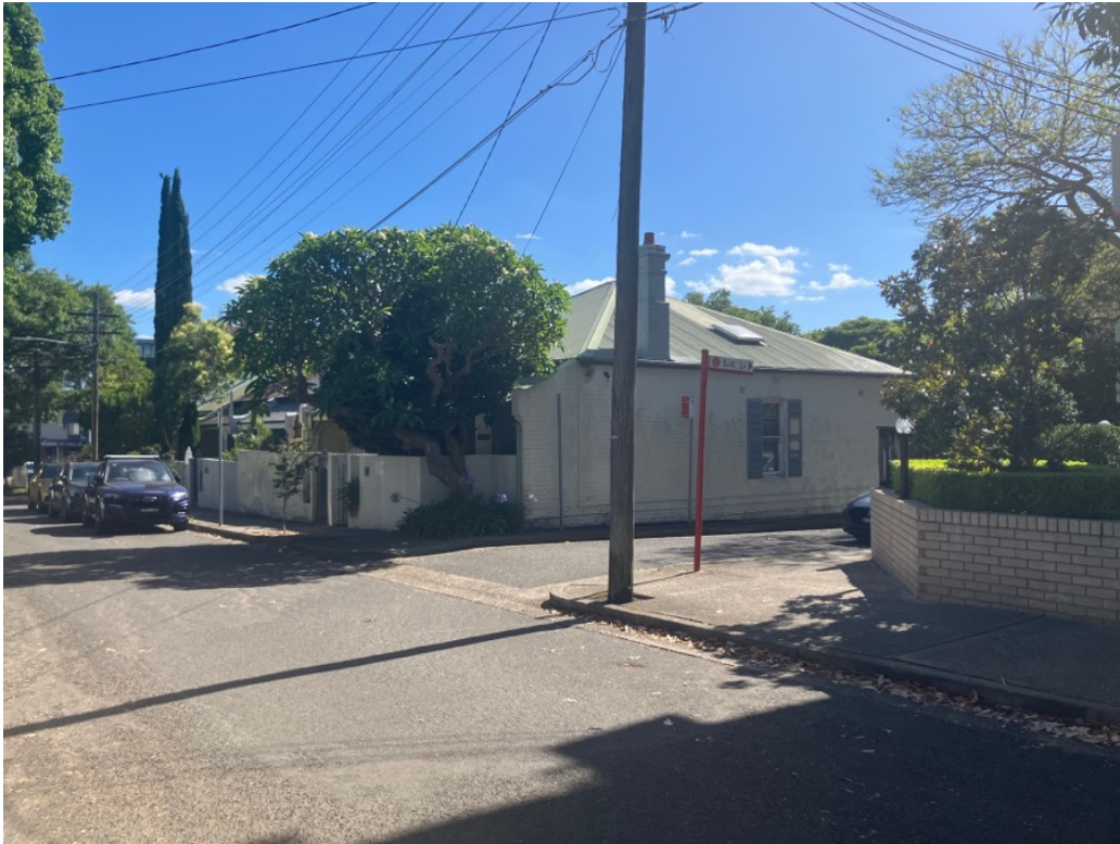
Figure 7: View looking north towards the group of cottages showing No. 27 Bydown Street addressing Olive Lane.
