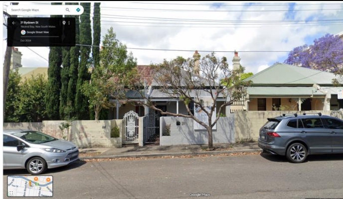
FIGURE 4: 33 & 31 Bydown Street Source – Google Street View 2024 image
