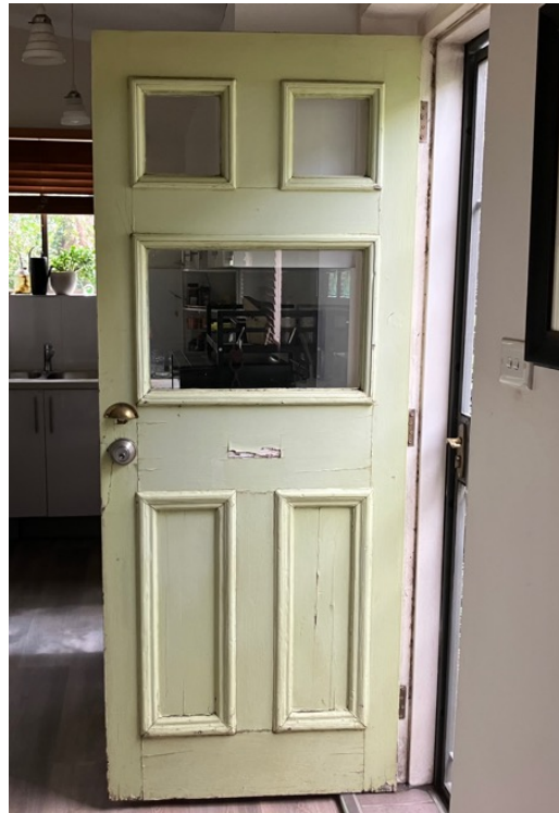
Figure 43: Original six panelled back door, modified to accommodate a glazed panel.
