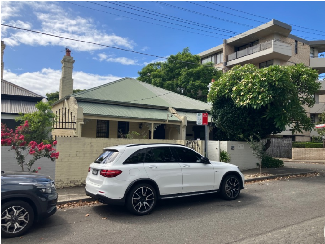
Figure 13: Streetscape presentation of No. 29 Bydown Street, the northern of the two semi-detached cottages.
