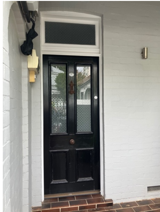
Figure 29: Front door of No. 31 Bydown Street showing original opening and fanlight.
