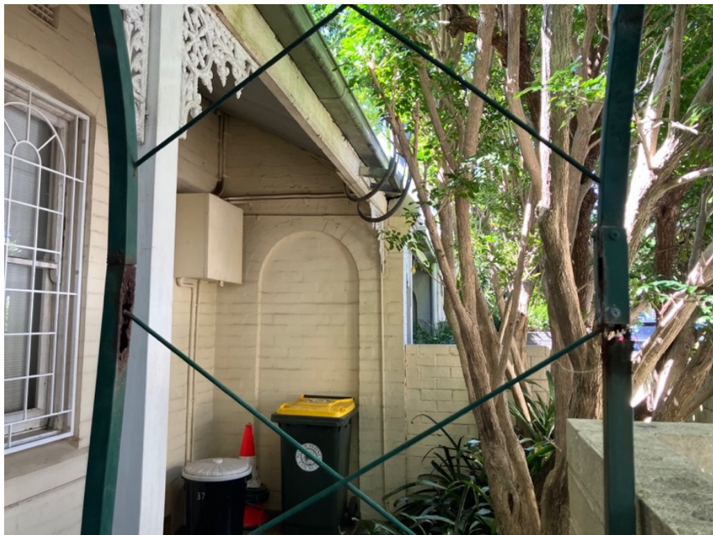
Figure 45: Front entrance verandah of No. 37 Bydown Street showing original form and fenestration and likely filigree wrought iron lacework, which exists at No. 29, 33, 35 and 37.
