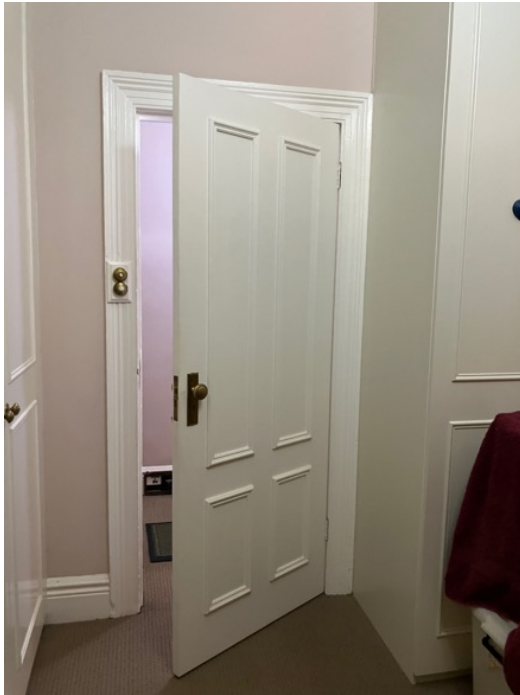
Figure 46: Likely original four panelled timber door, architraves, and skirtings.
