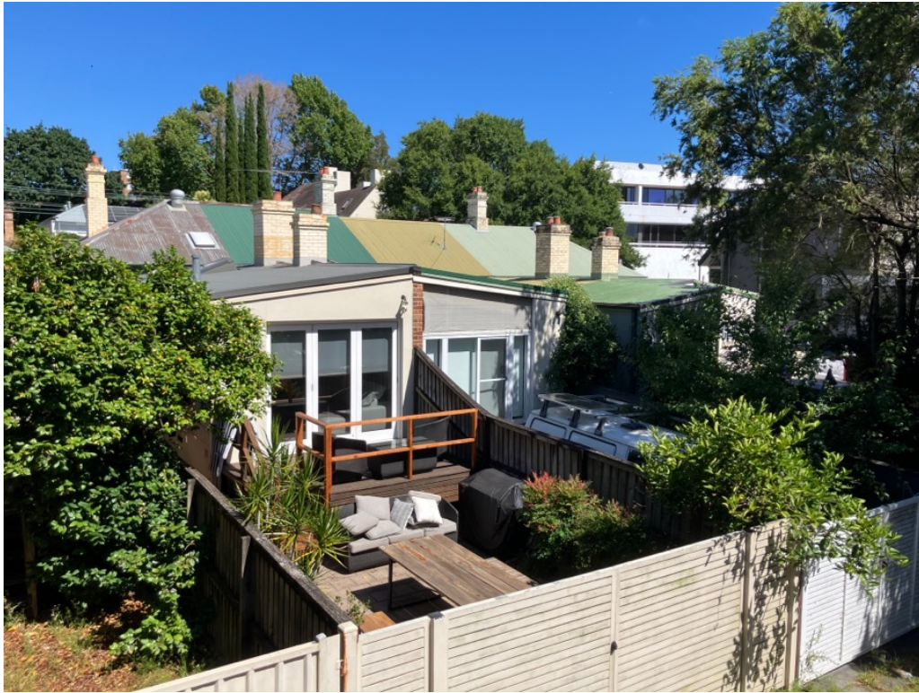
Figure 15: View of the rear of the row of four including No. 31-37 inclusive, looking north-west.
