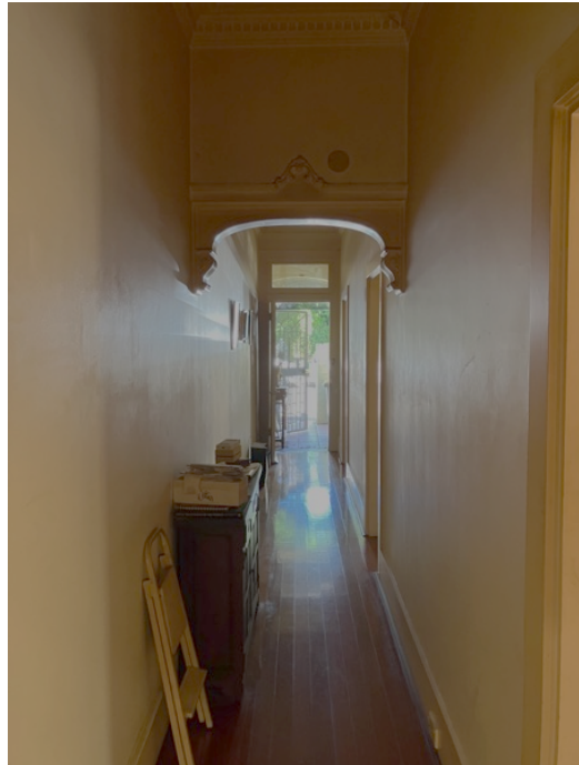
Figure 24: Internal hallway of No. 29 Bydown Street in its original configuration including its relationship to rooms and front door fanlight.
