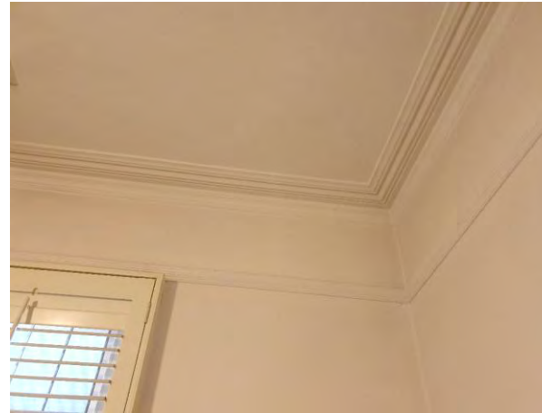
Bedroom 1 - Cornice and picture rail
