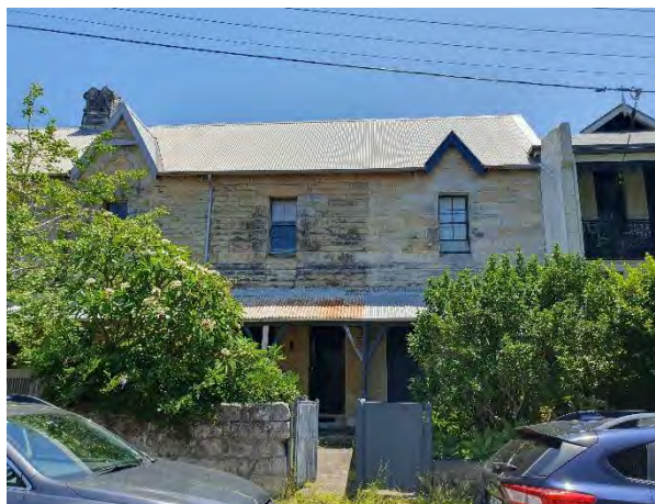
Northern extent of terrace group (#22 end)
