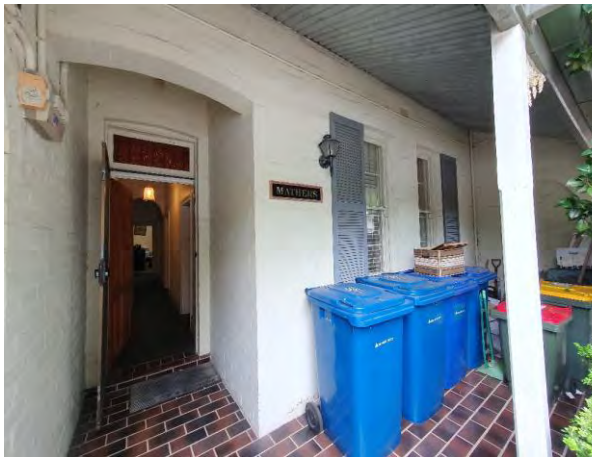
Front elevation – set in entryway, double timber sash windows, simple timber column holding up verandah, corrugated sheeting on verandah
