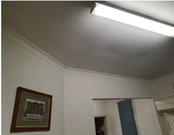
Rear portion of the cottage – contemporary cornice
