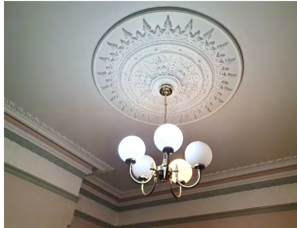
Bedroom 1 – ceiling rose, cornice, picture rail– all non-original, added
