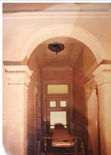
Entry corridor - during renovations
