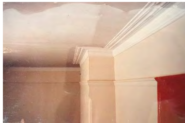
Ceiling and cornice – before renovations
