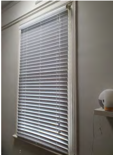
Bedroom 1 – timber sash window
