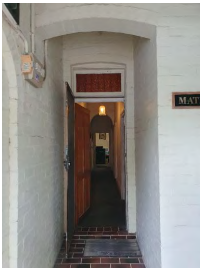
Recessed entry way, security door, main door and transom light
