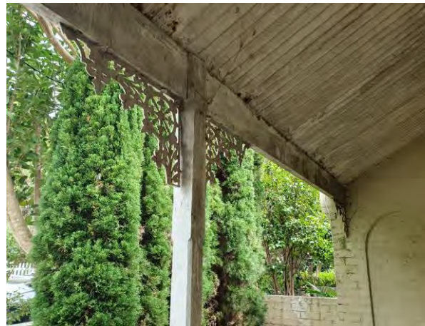
Simple timber column holding up verandah, filigree, corrugated sheeting on verandah
