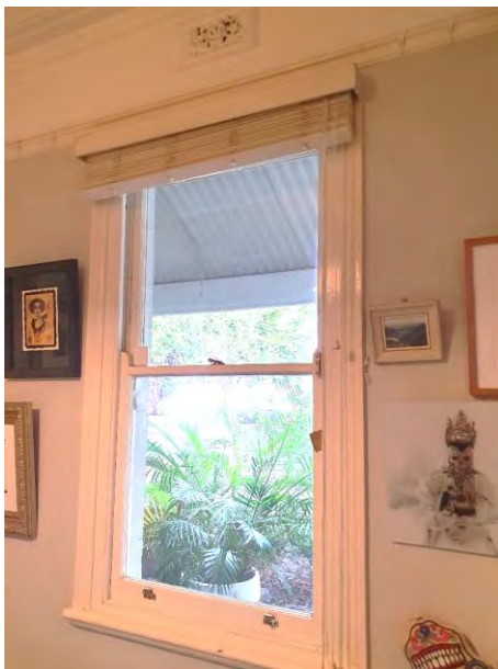
Bedroom 1 - single timber sash window
