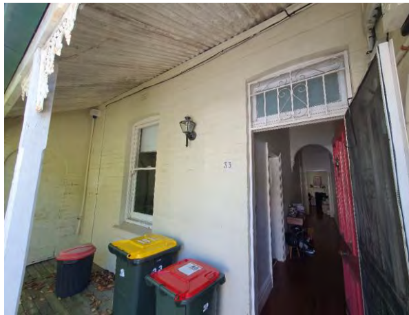
Front elevation – single timber sash window, simple timber column holding up verandah, filigree
