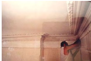
Installation of new decorative cornices
