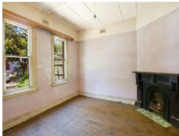
Interior of 84 Parraween Street showing more decorative fireplace and timber batten ceiling. (Source: https://www.realestate.com.au/property/84-parraween-st-cremore-nsw-2090/ )
