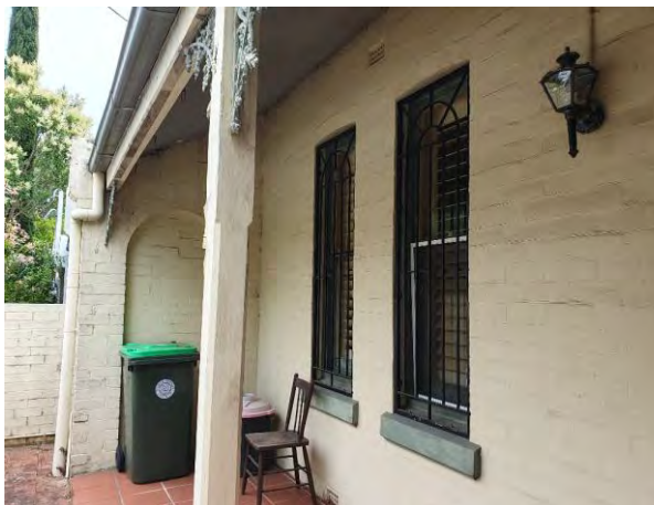
Front elevation – double timber sash windows, simple timber post and beam supporting verandah, filigree, corrugated sheeting on verandah
