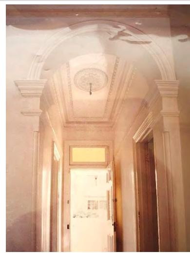
Entry corridor – after renovations. Note decorative cornice, ceiling rose, archway
