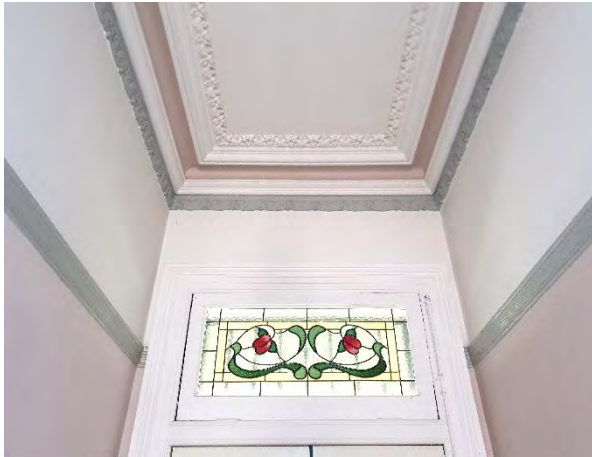
Entry corridor – transom window, picture rail, cornice – all non-original, added
