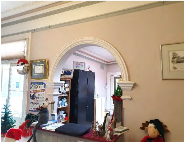
(Non-original, added) Archway into rear portion of cottage
