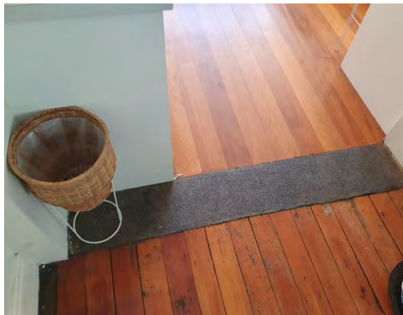
Threshold between original floorboards (bottom) and new floorboards (top)
