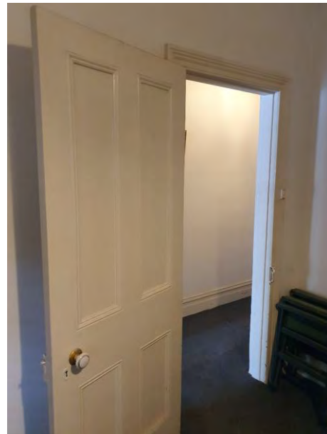
Bedroom 1 - Door and architrave
