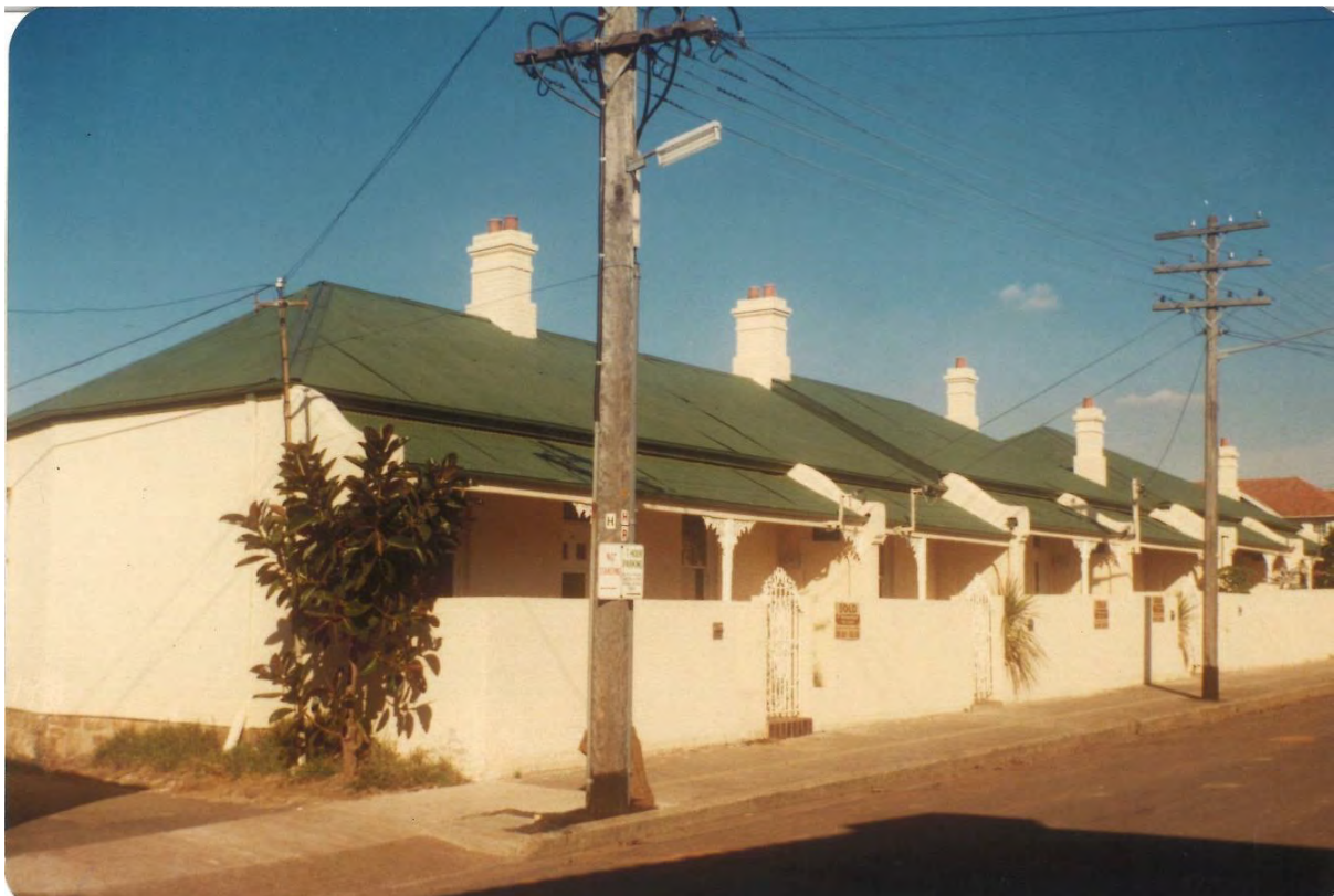
Figure 4 1980 photograph of the subject properties (looking south with No. 37 in the foreground) – after the construction of the 1.8m front fence across all the properties, roof changed and brick painted. (Source: Stanton Library, Call Number: LH REF CT 12/8.)
