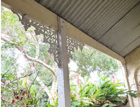
Verandah – timber post, beam and filigree
