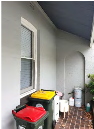
Entry porch – single timber sash window
