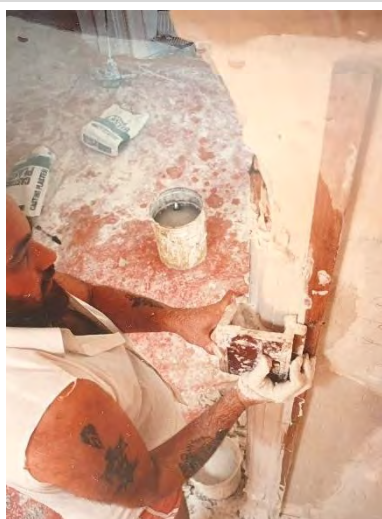
Plasterer scribing edge under entry corridor archway
