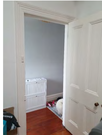
Bedroom 1 – timber door and architrave
