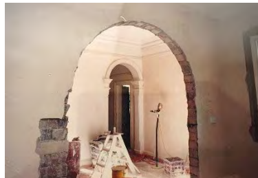
Archway during renovations
