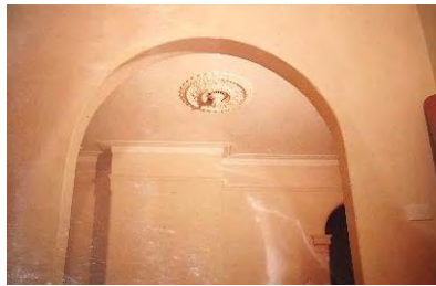
Archway before renovations
