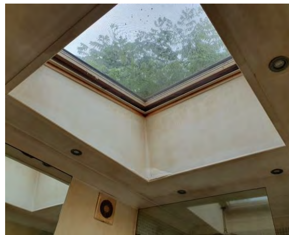
Skylight in bathroom
