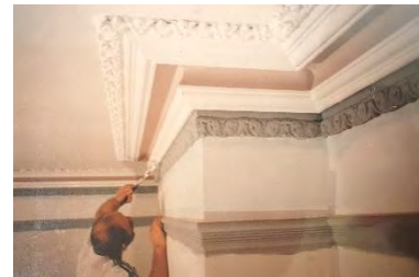
Painting of decorative cornices
