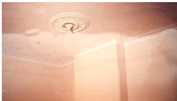
Original ceiling rose and cornice – before renovations
