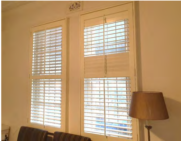
Bedroom 1 - Double timber sash windows
