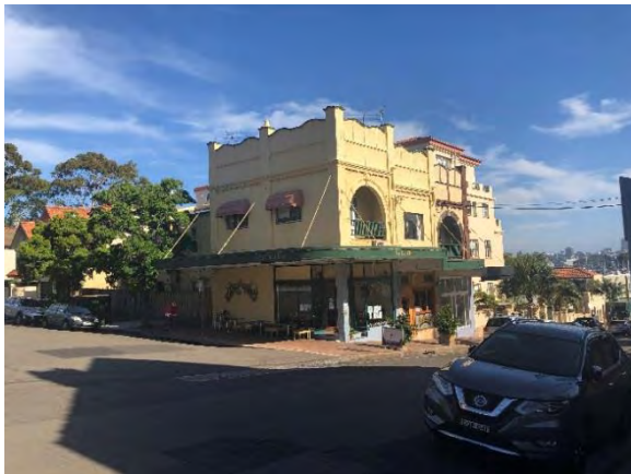
Figure 5.22 11–15 Hayes Street. (Source: GML, 2018)
