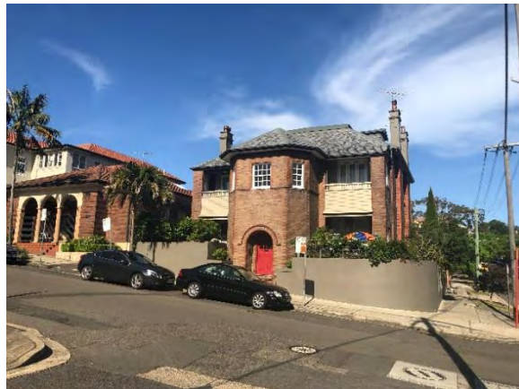
Figure 5.23 17 Hayes Street. (Source: GML, 2018)
