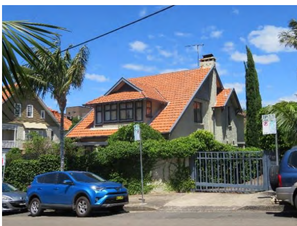
Figure 3.3 8 Hayes Street. (Source: GML, 2018)
