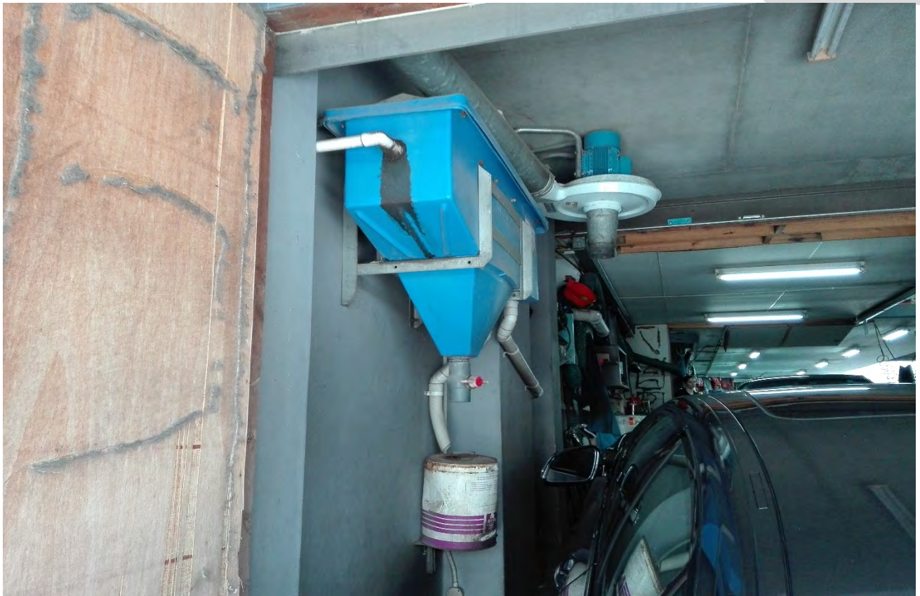
Plate 7: Oil separator AST located at 31 Atchison Street.
